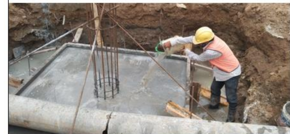
West side solar parking footing curing work
