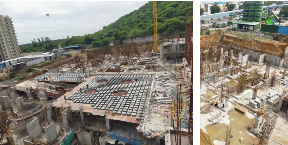
Figure 9 Site progress photo
