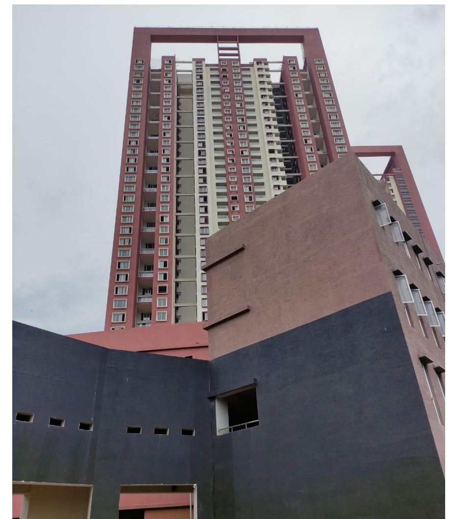
VIEW OF APARTMENT RESIDENTIAL BLOCK FROM
