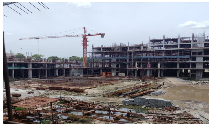
WEST WING ON-GOING CONSTRUCTION (MOI)
