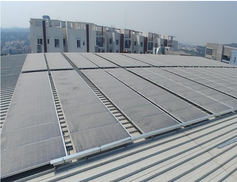
SOLAR PANEL INSTALLATION
