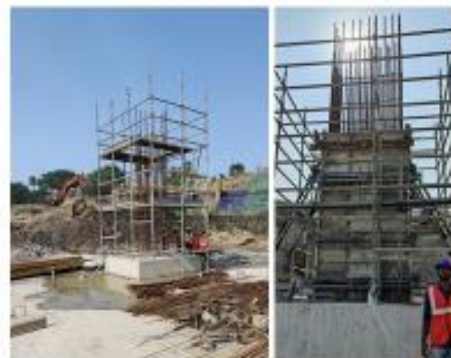
COLUMN SHUTTERING AND REINFORCEMENT
