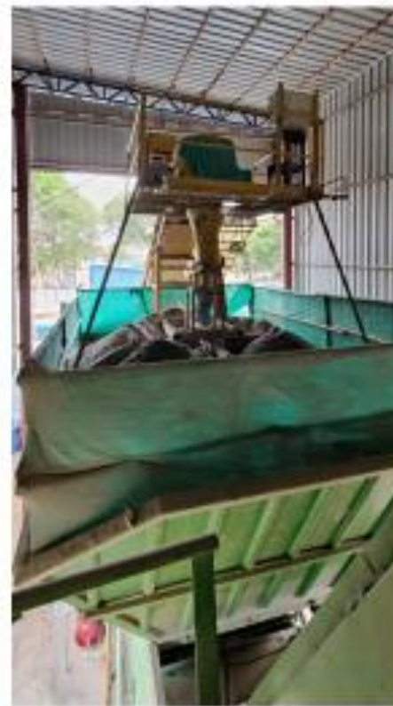
Aggregates gets collected in the tank
