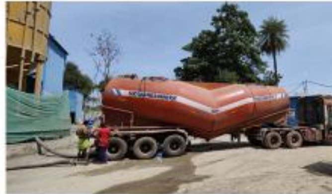
Filling of silos with cement
