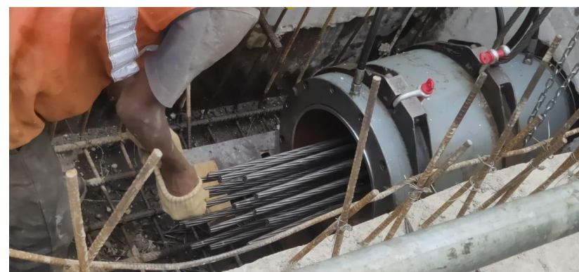
POST TENSIONING OF TENDONS AT SITE
