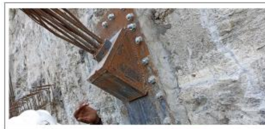
ANCHORING AT SITE
