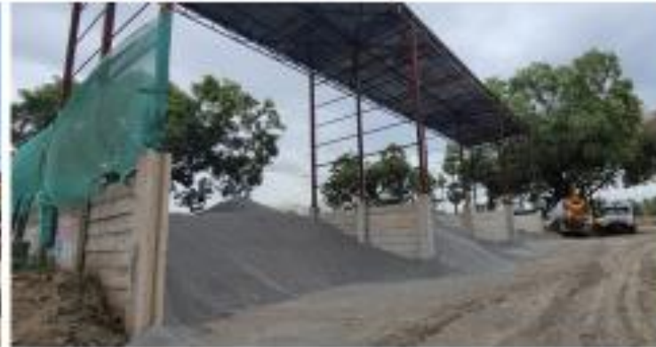
Aggregates storage yard
