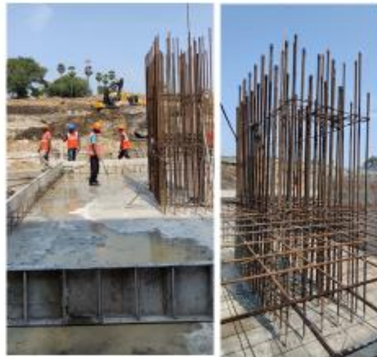
REINFORCEMENT AND SHUTTERING OF RAFT FOUNDATION
