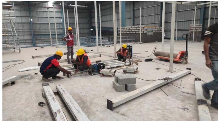
Interior fitout project
