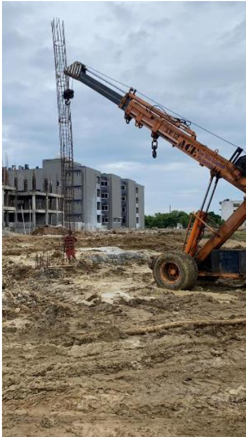
Placing reinforcement
