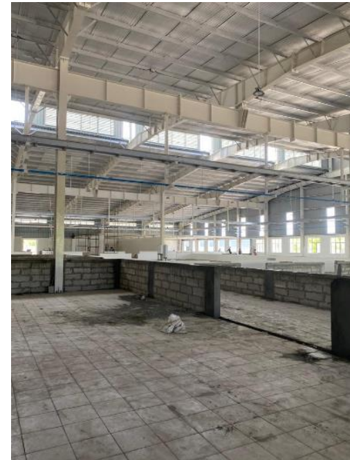
partition wall work
