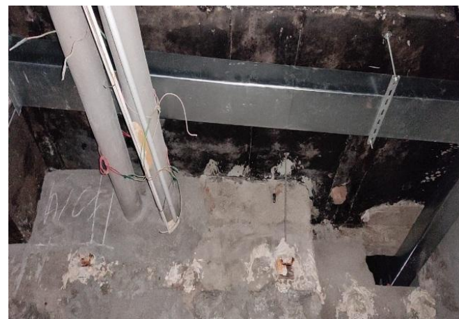
Duct work in progress at toilet area
