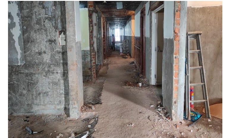
Demolishing WIP target
