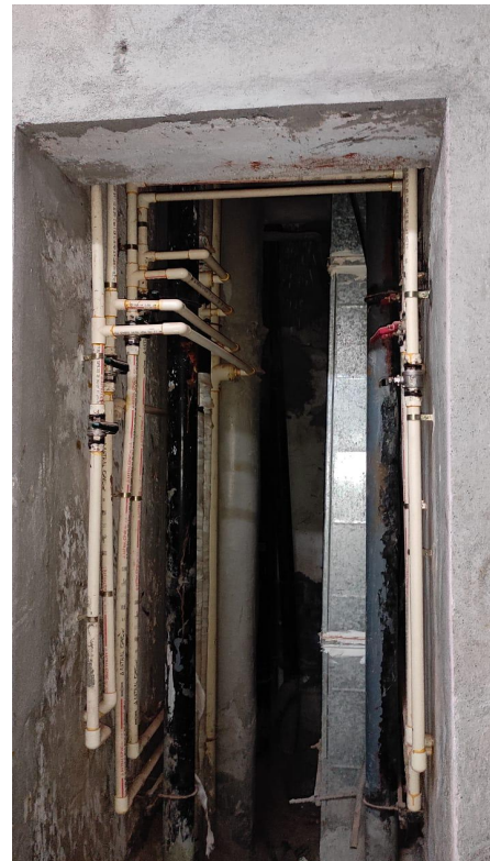
Plumbing pipes alignment Mock up done for roll over work
