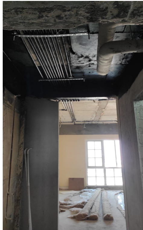
10 rooms MS conduiting Work completed
