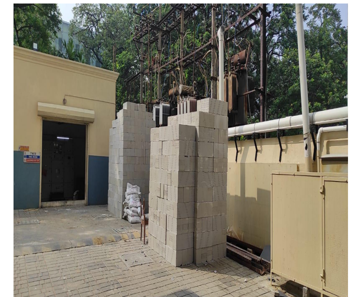
Aerocon Block received for the 19 th floor Civil work
