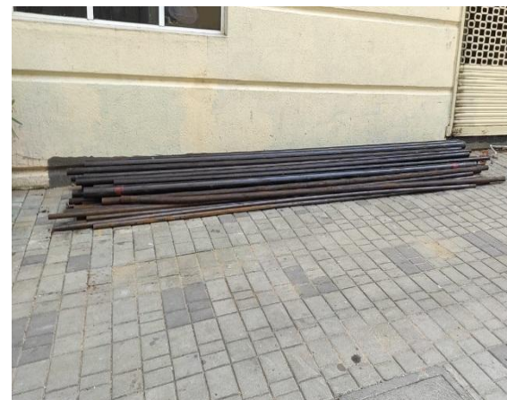
MS Pipe received for 18 th floor fire line work
