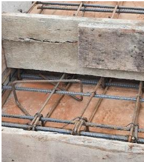
Placement Of Tension Rods In Each Staircase To Avoid Bending Due To Compression
