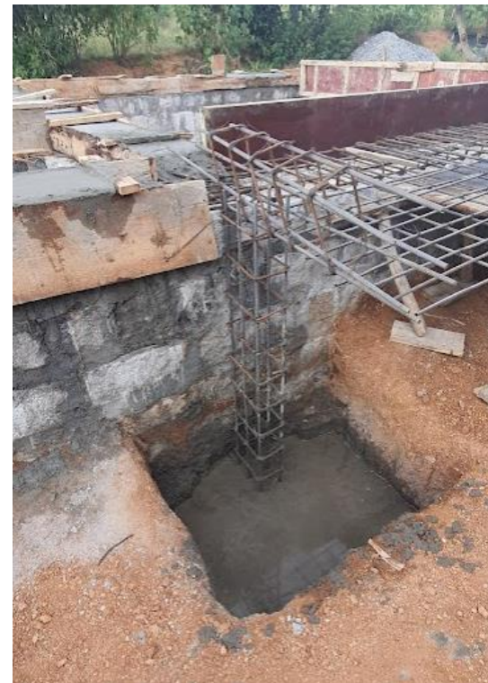
TYPICAL SECTION OF EXENTRIC FOOTING WITH RUBBLE FOUNDATION
