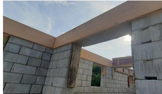
SHUTTERING FOR LINTEL ON DOOR OPENINGS
