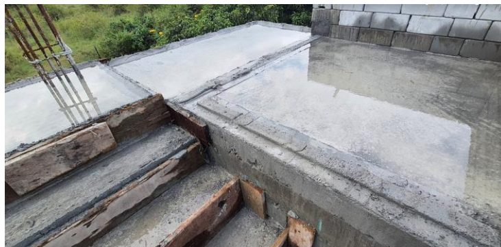
AFTER CONCRETE CASTING SLAB LEFT FOR CURING BY PONDING
