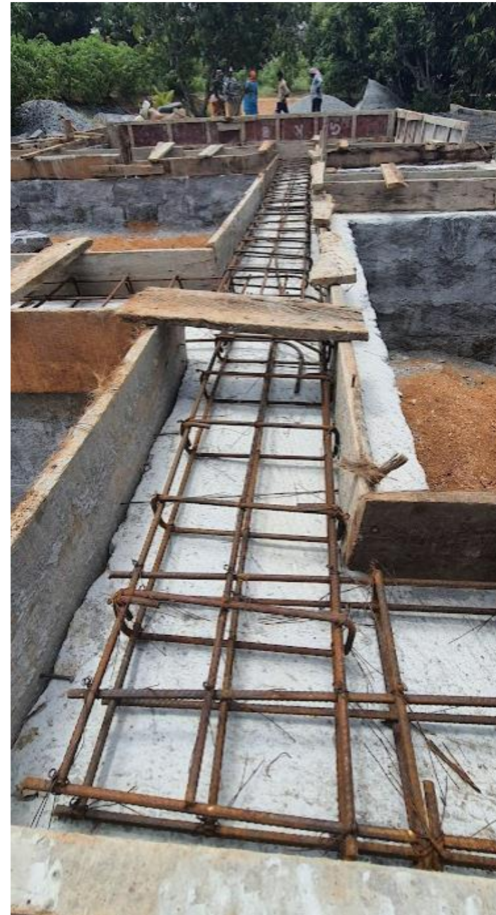
SHUTTERING FOR CONCRETE CASTING
