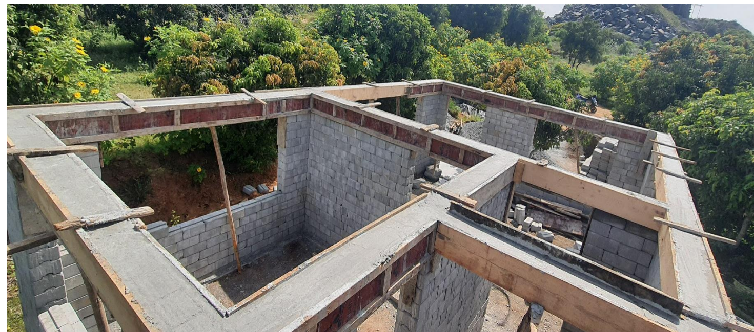
SHUTTERING FOR LINTEL BEAM ON WALLS
