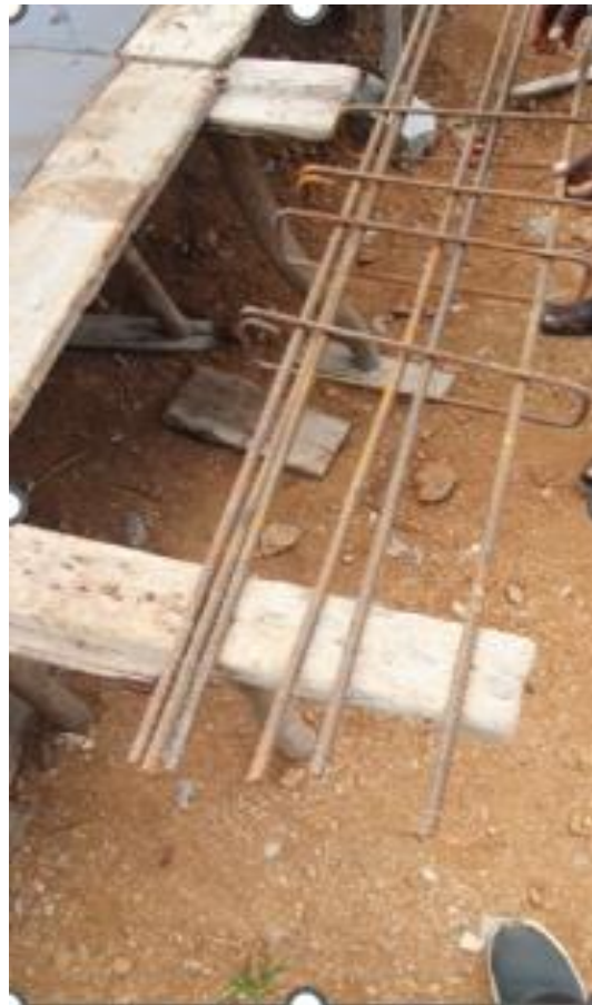
TIEING OF REINFORCEMENT WITH STIRRUPS
