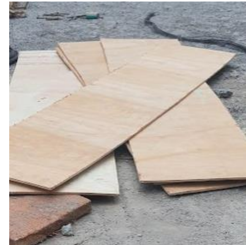
Plywood's Are Placed Over Centering To Get Neat Finish While Casting
