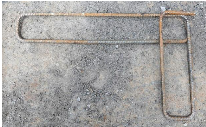
8mm TMT Rod Is Bended To Make Module
