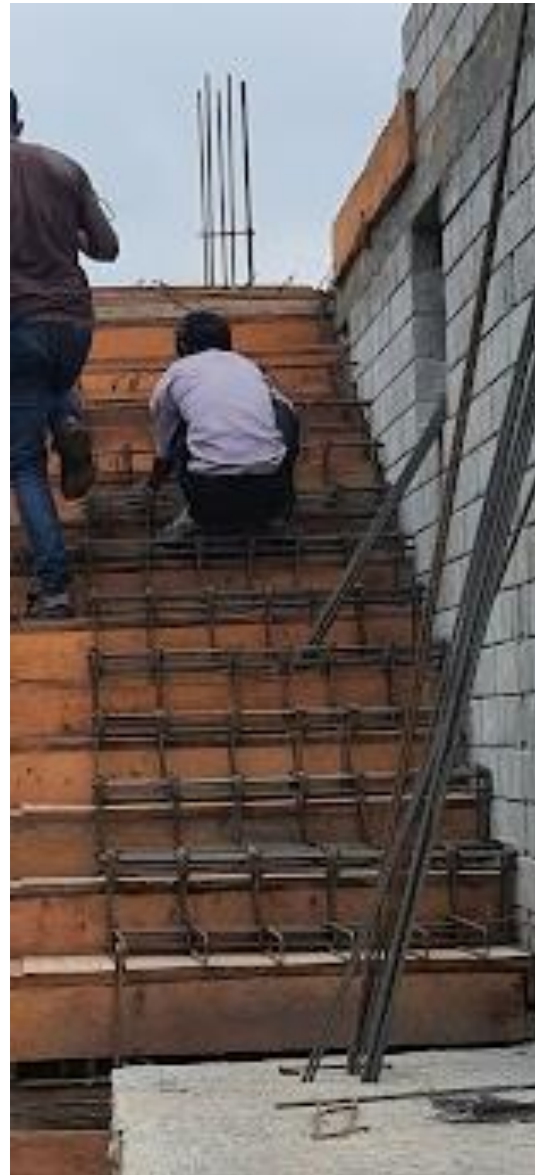
Tieing Of Reinforcement For Stairs
