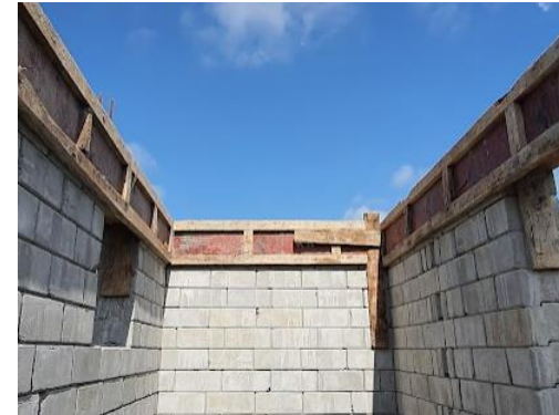
SHUTTERING FOR LINTEL BEAM ON WALLS
