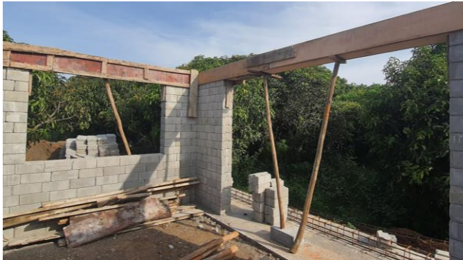
SHUTTERING FOR LINTEL AT LARGE OPENINGS WITH SUPPORTED BY CASURINA POLES
