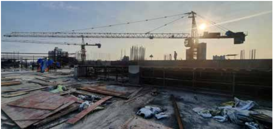
Cranes used for the transportation of concrete
