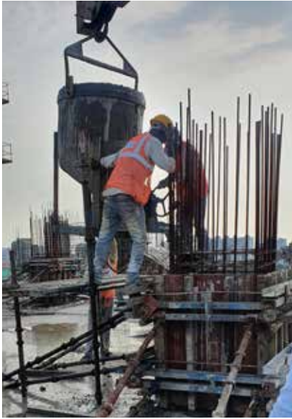
Cranes used for the transportation of concrete
