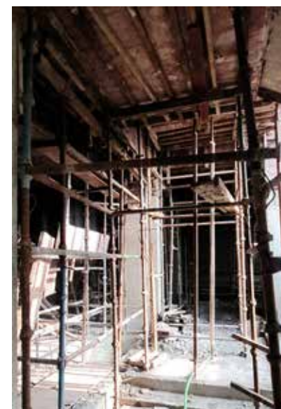
H Shuttering frames which is made of mild steel to keep the shape of concrete .
