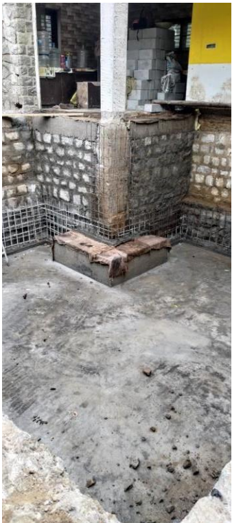
JACKETING DONE FOR THE COLUMN TO INCREASE THE SIZE OF THE COLUMN
