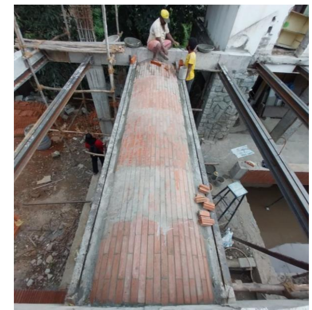
Step 5: Keeping the overlap, lock the formwork in place with the wedge Step 6: continue to arrange the bricks in the form of a vault
