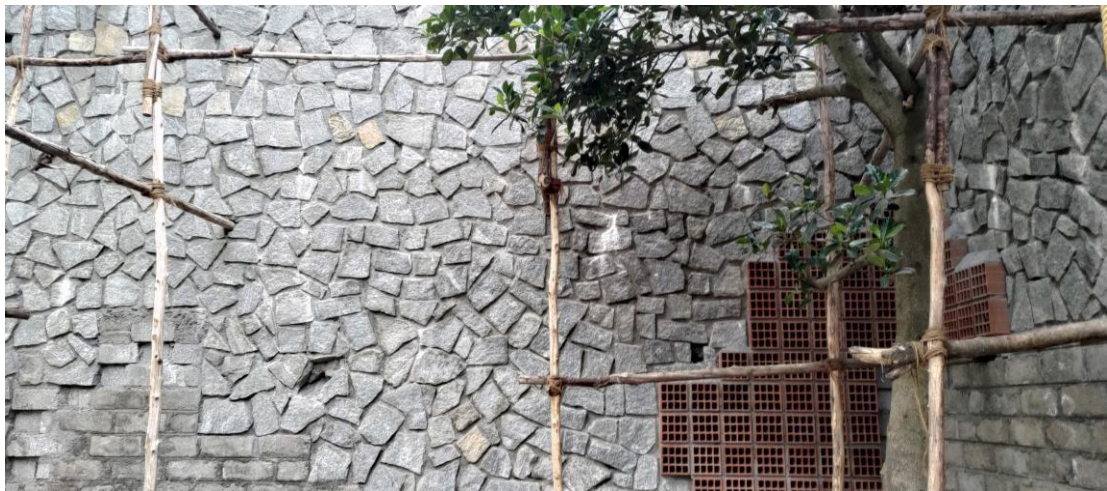
COMPOSITE STONE MASONRY WALL
