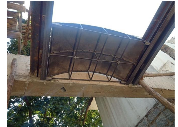
Step 1: Keep the formwork in place on the L- angle with the wedge
