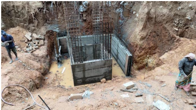
CONCRETING DONE FOR LIFT SHAFT
