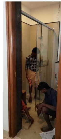
GLASS FIXING FOR THE PARTITION OF WET AND DRY AREA IN BATHROOM
