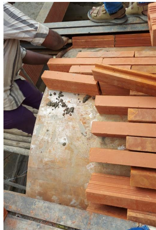
FABRICATION OF FORM WORK
