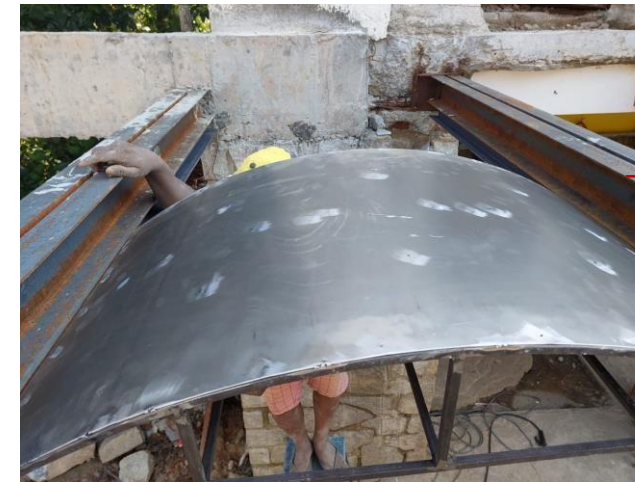
Step 1: Keep the formwork in place on the L- angle with the wedge
