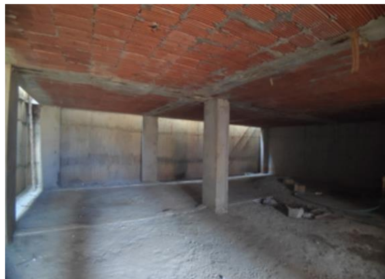
FILLER SLAB IN BASEMENT
