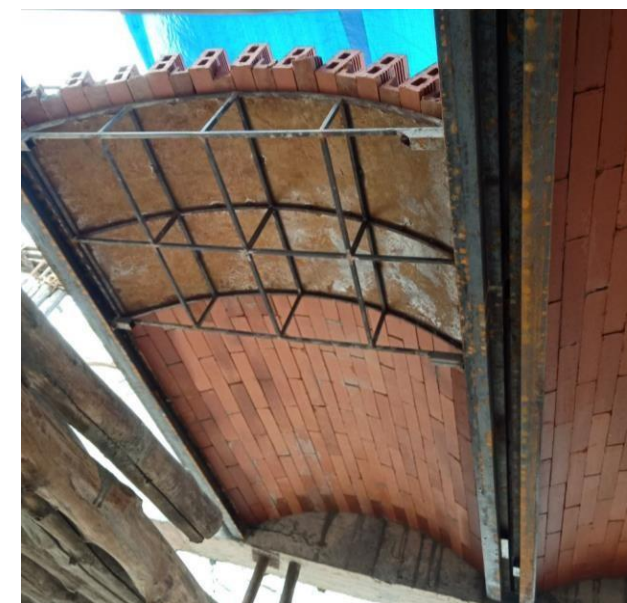
Step 5: Keeping the overlap, lock the formwork in place with the wedge Step 6: continue to arrange the bricks in the form of a vault
