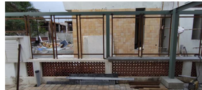
RODS ARE WELDED FOR GABION WALL
