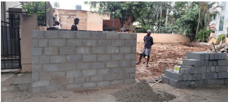
TEMPORARY SHELTER FOR WATCHMEN
