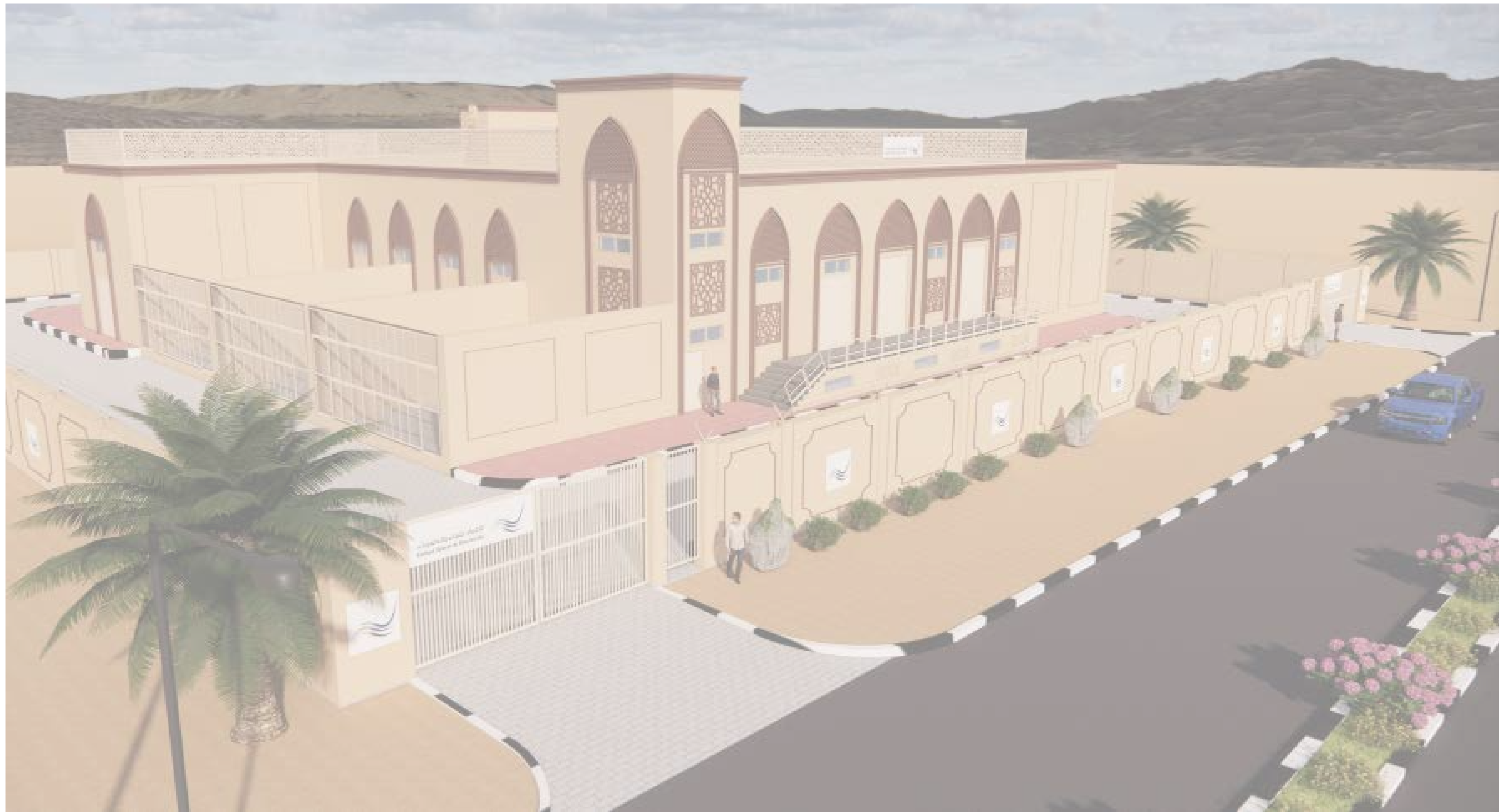
PROJECT 1: AL AQAH SUBSTATION
