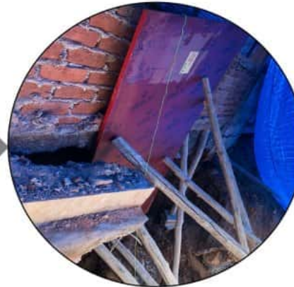
Supports are provided to avoid more snag and the building to collapse
