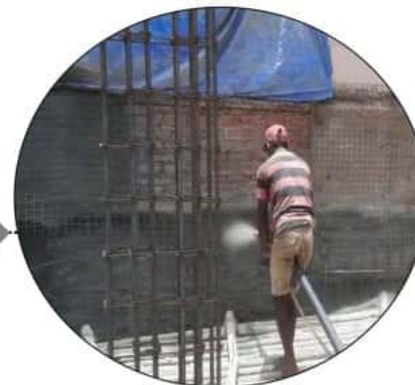
Applying concrete proposed at high velocity primarily on the vertical surface. It is a mortar or high-performance concrete conveyed through a hosepipe and pneumatically shot at high force at the back surface.
