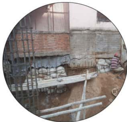
The gap is covered with soil filled bags ,then supported with iron rods which holds grip from underneath and later covered
