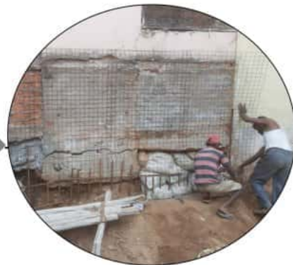
The gap is covered with soil filled bags ,then supported with iron rods which holds grip from underneath and later covered
