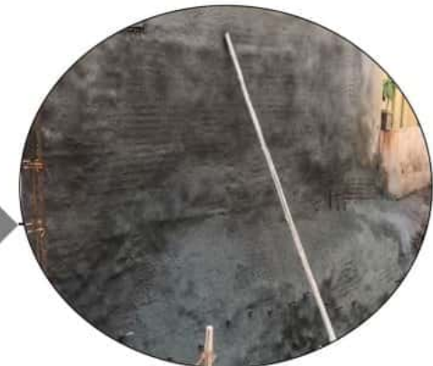
Applying concrete proposed at high velocity primarily on the vertical surface. It is a mortar or high-performance concrete conveyed through a hosepipe and pneumatically shot at high force at the back surface.
