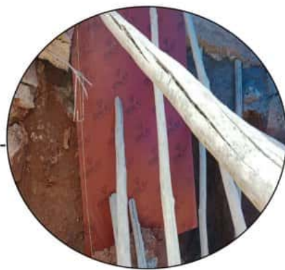
Supports are provided to avoid more snag and the building to collapse
