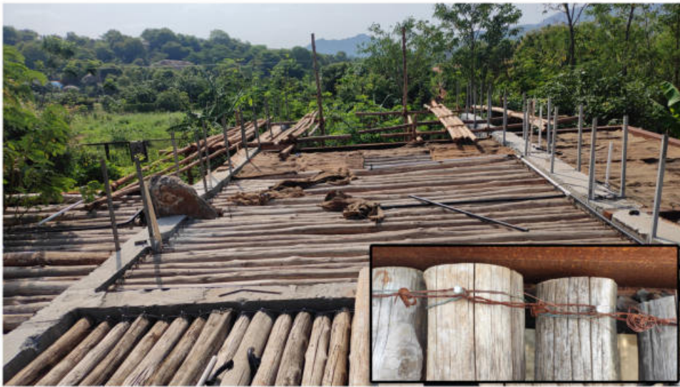
Public spaces were covered with causerina and private spaces are covered with casurina poles along with RCC.
