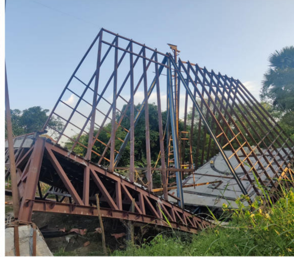
Horizontal 4"x2" Box section supports installation along with wooden reapers.
