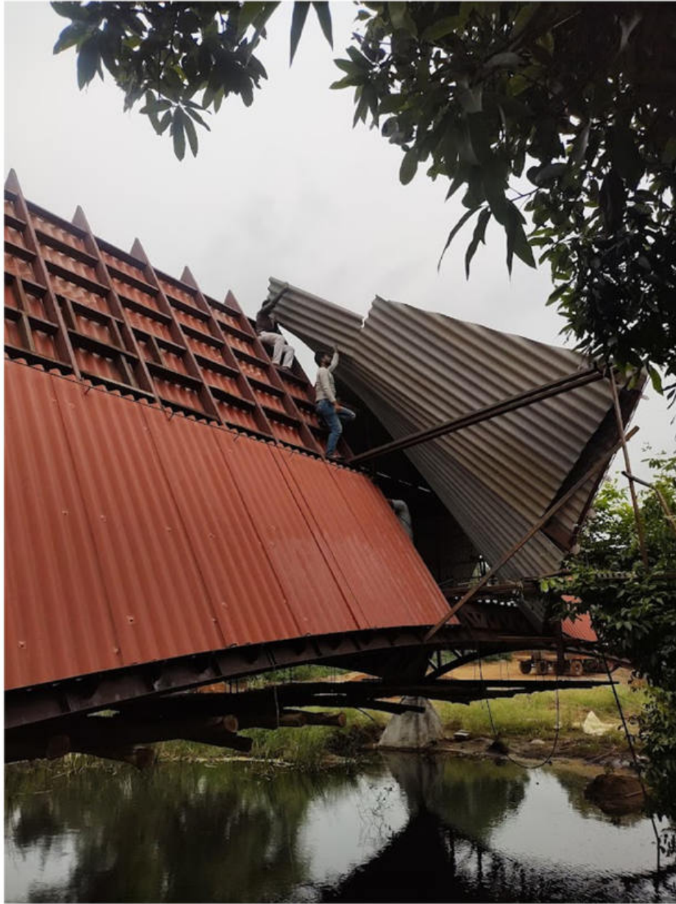
Structure opening for entrance
