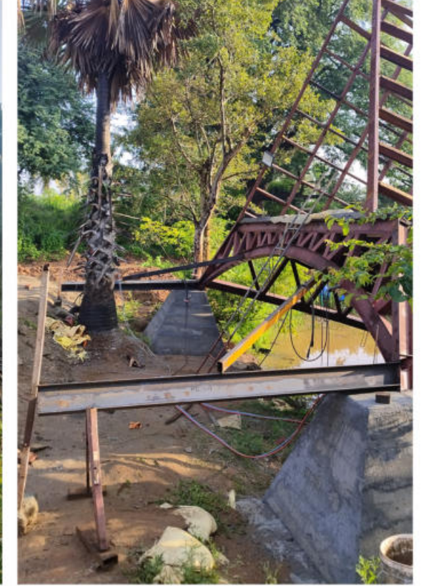
I- Beam structure extension
