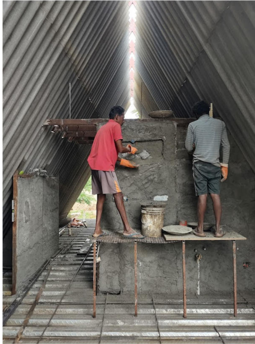
Partition wall plastering
