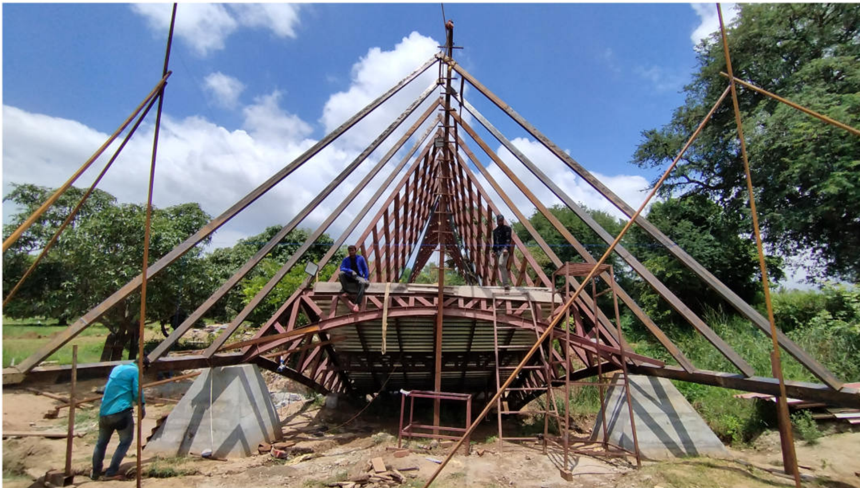
Vertical 6"x2" Box section supports installation.
