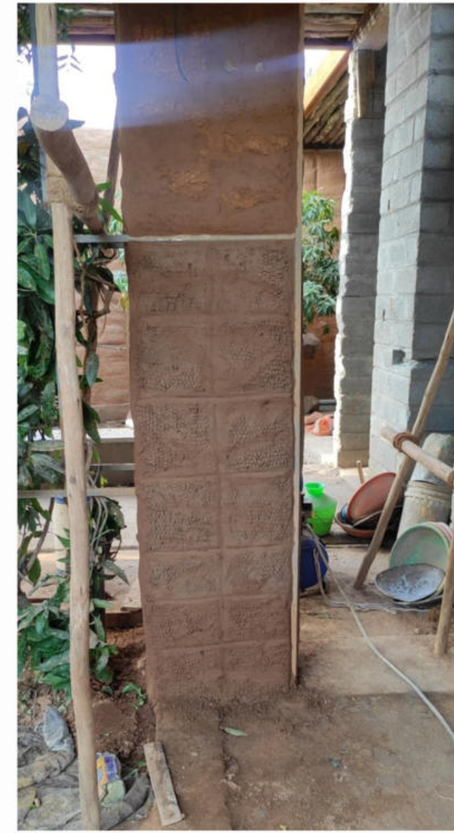
Waterproofin paint coating were applied to the poured earth wall surface.
