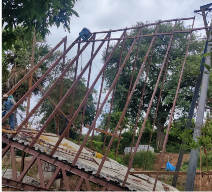
Vertical 6"x2" Box section supports installation.
