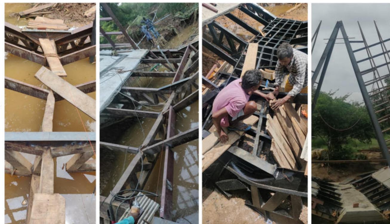
Center foundation construction process
