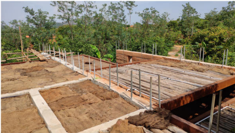
Layer of jute were laied above the casuarina.
