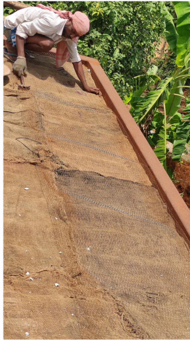
Chicken Mesh were laied above jute.
