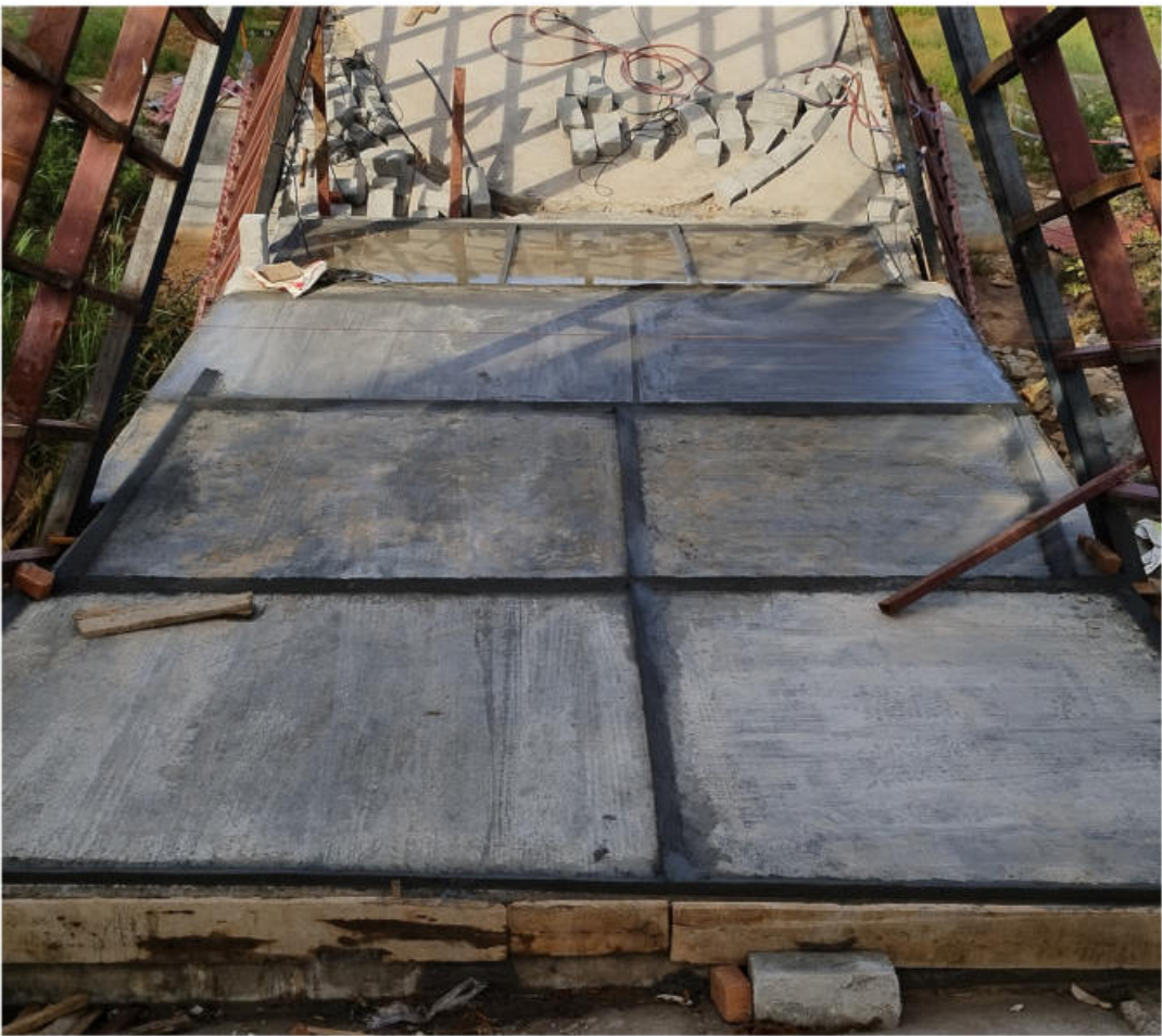
6cm thick living room slab is been created above the box section
