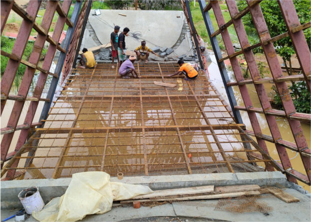
Box section were welded and chicken mesh is laied and tied using binding wires by masons.
