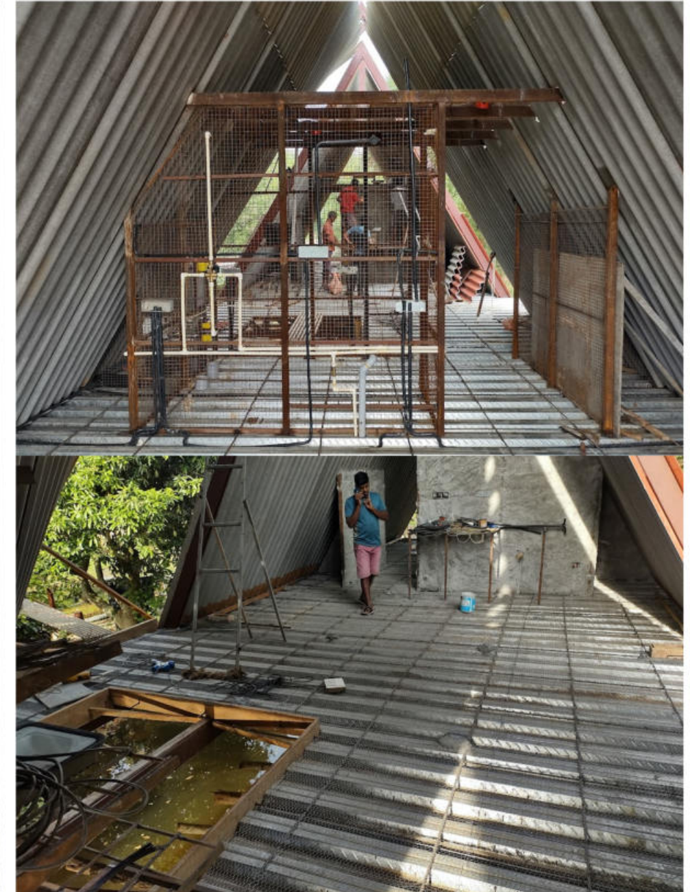
Partition wall welding and pond opening view.
