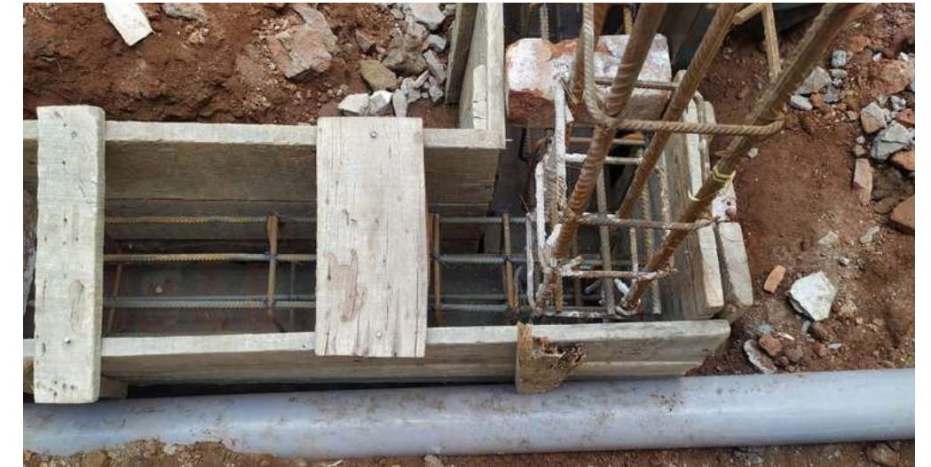
Plinth level construction
