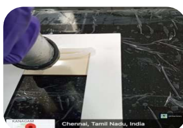
Fig 4.5 Application of sealants
