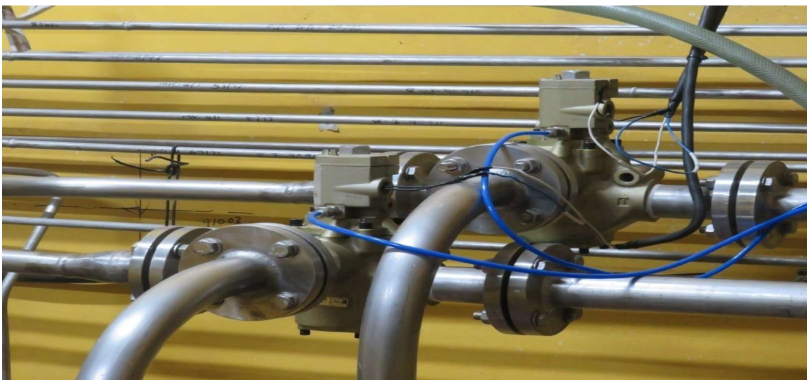
Fig: 4.8: Three-Way solenoid valve (Ross valve)
