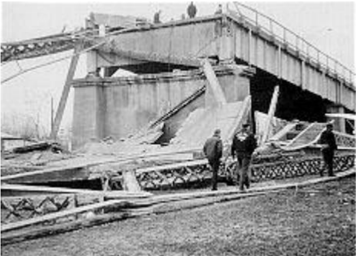
Fig 1.6. The collapsed Silver Bridge
