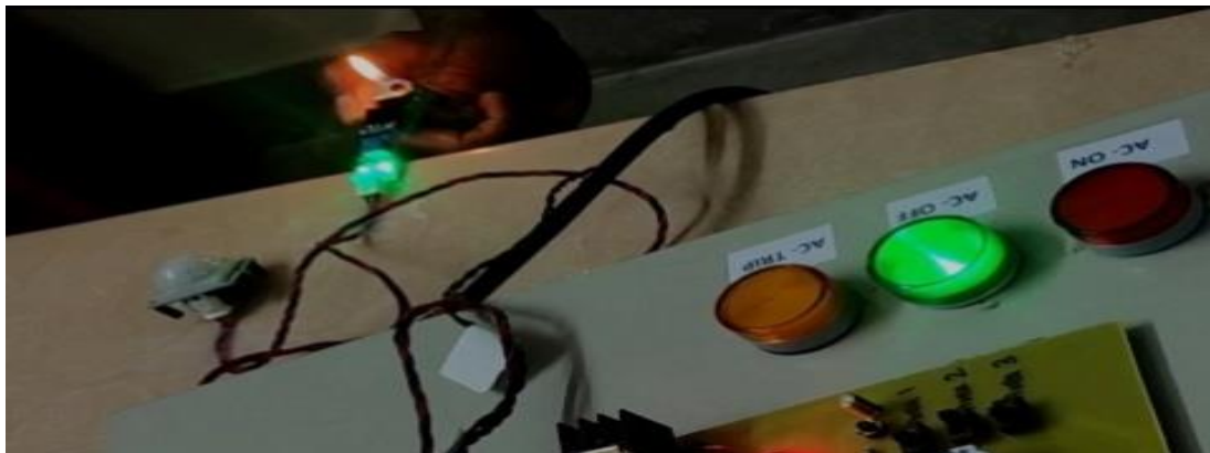
Figure 29 Fire sensor activated by naked fire
