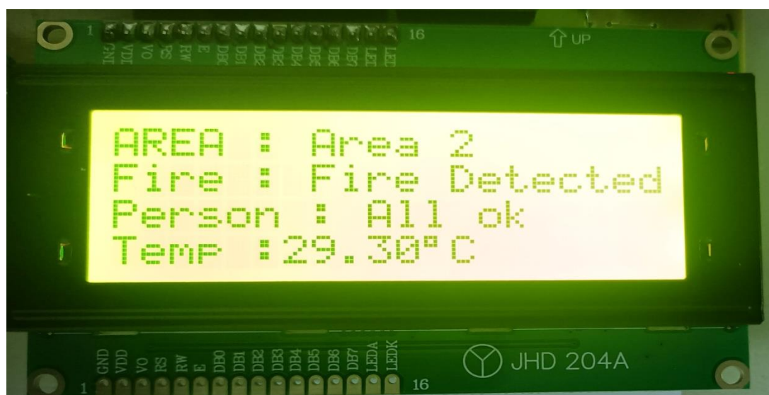
Figure 30 LCD shows fire detected in IOT module
