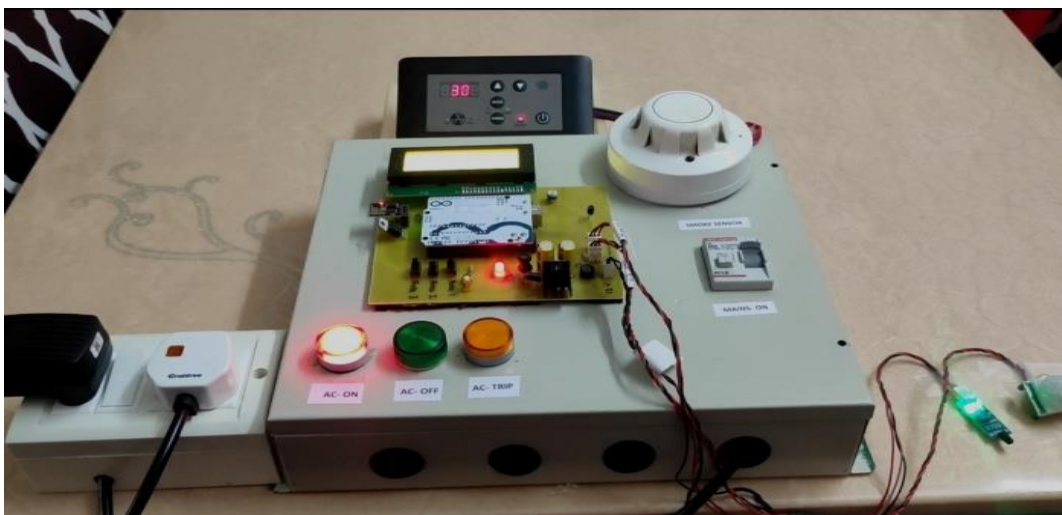
Figure 27 AC compressor switches ON after 3 minutes
