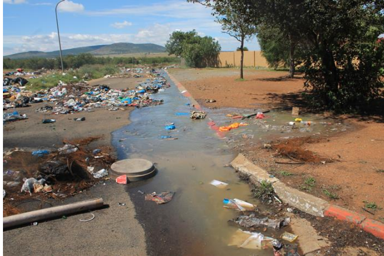
Figure. 1.1: Sewage leakage
