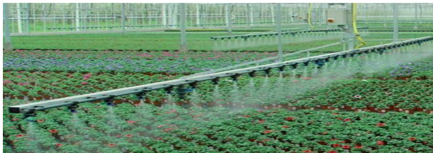
Fig:1.3 : Sprinkler Irrigation System
