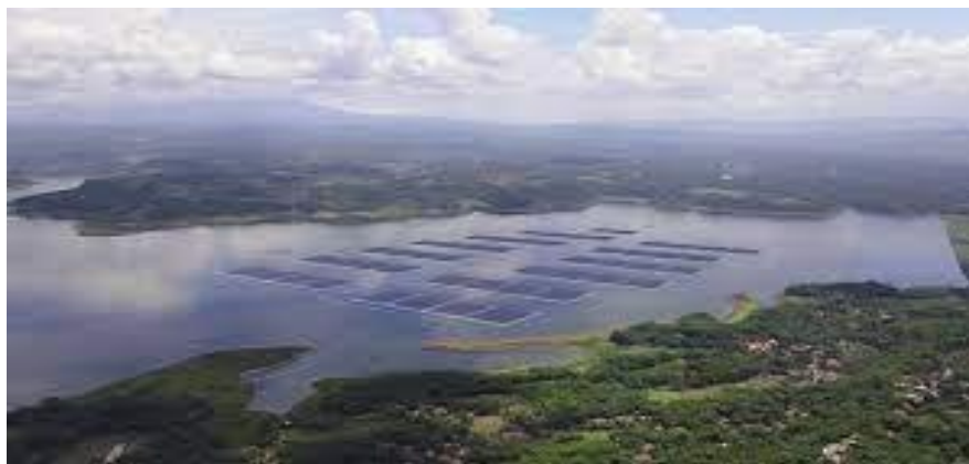
Fig 2.2: Citrate Reservoir Floating Photovoltaic
