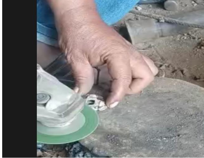
Fig: 4.4 grinding process of the welded part
