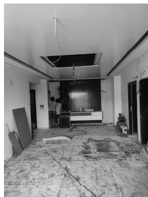
TV UNIT WALL CLADDING
