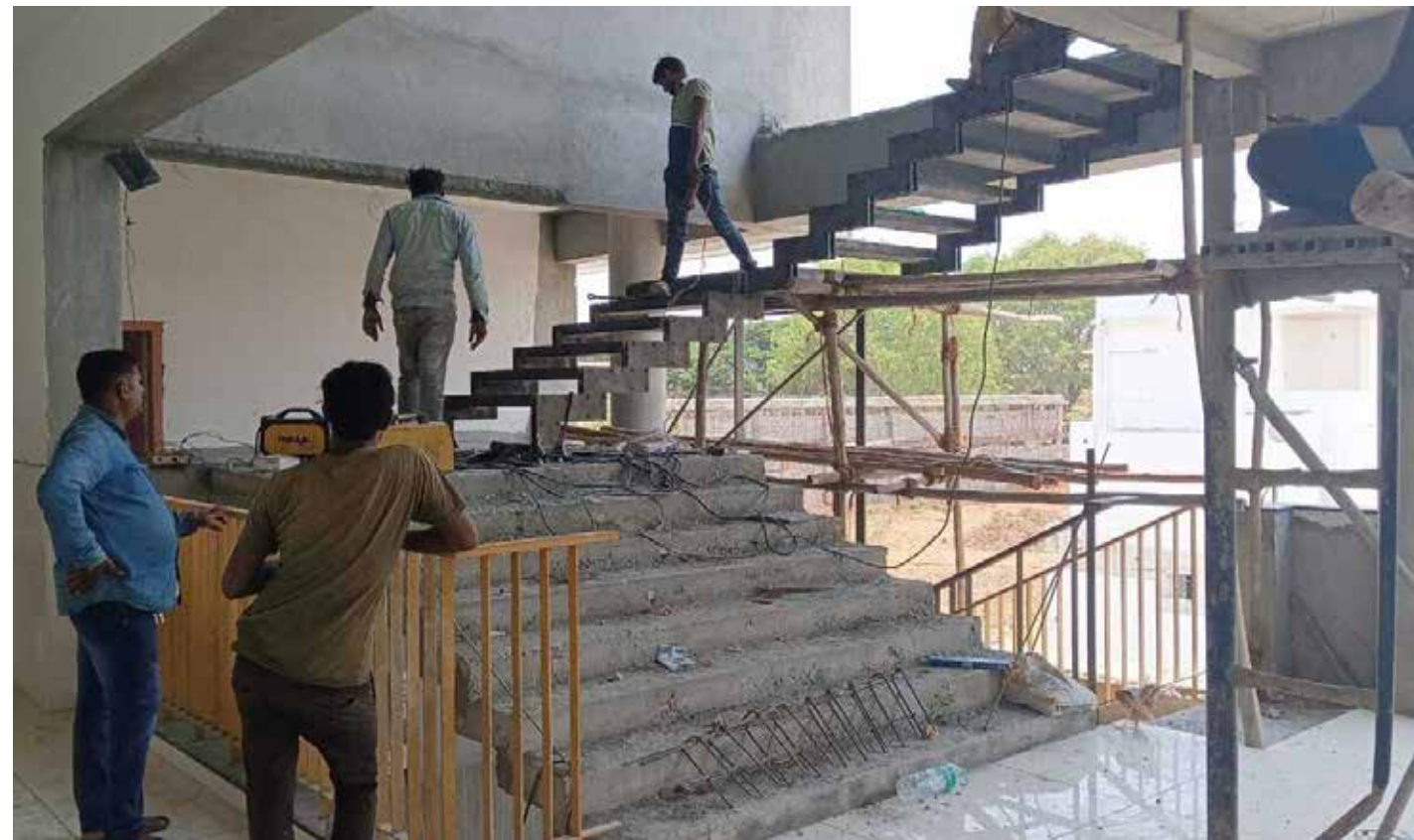
EXECUTION ON SITE
