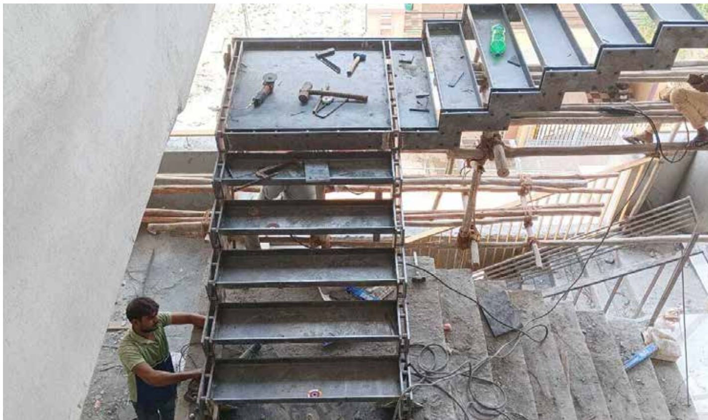
MS STAIRCASE FABRICATION
