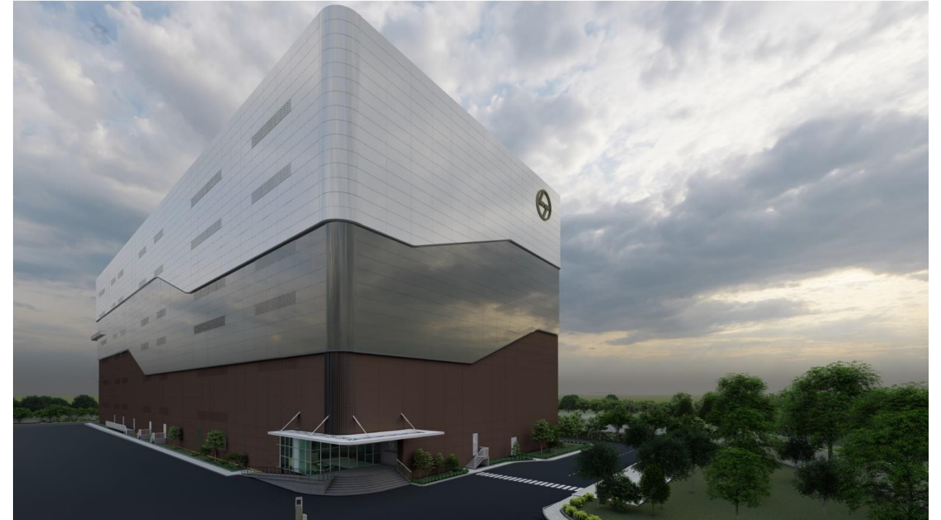
Option 2 – 300 mm projection in glazing and 600 mm projection in ACP
