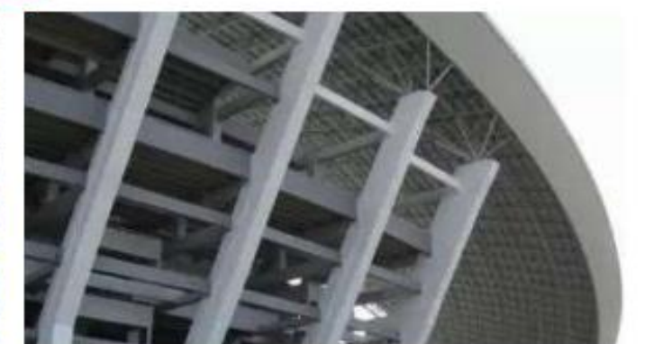
4 INCLINED COLUMNS –PAINT FINISH
