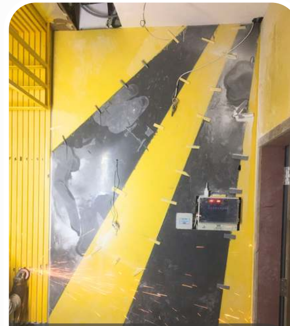
CORIAN LAMINATES CUT TO REQUIRED DIMENSIONS AND ATTACHED TO THE PLY BEHIND
