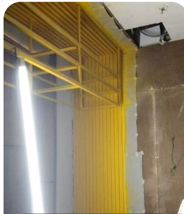
INSTALLED FLUTED PANEL, FINISHED WITH SPRAY PAINT IN THE COLOUR CHOSEN
