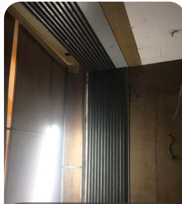
INSTALLATION OF FLUTED PANEL ( METAL PIPES)- WALL TO CEILING
