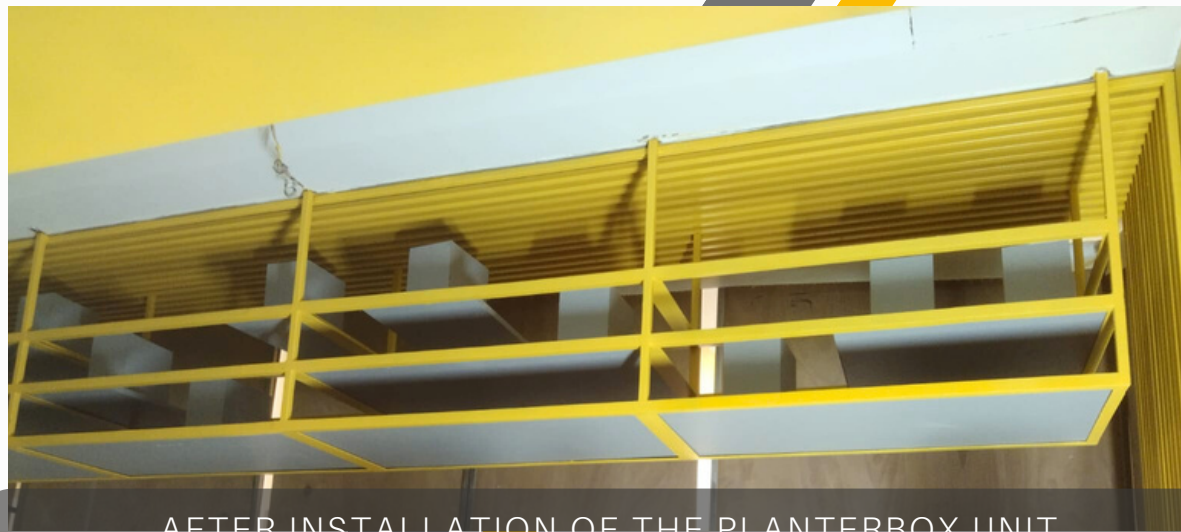
AFTER INSTALLATION OF THE PLANTERBOX UNIT
