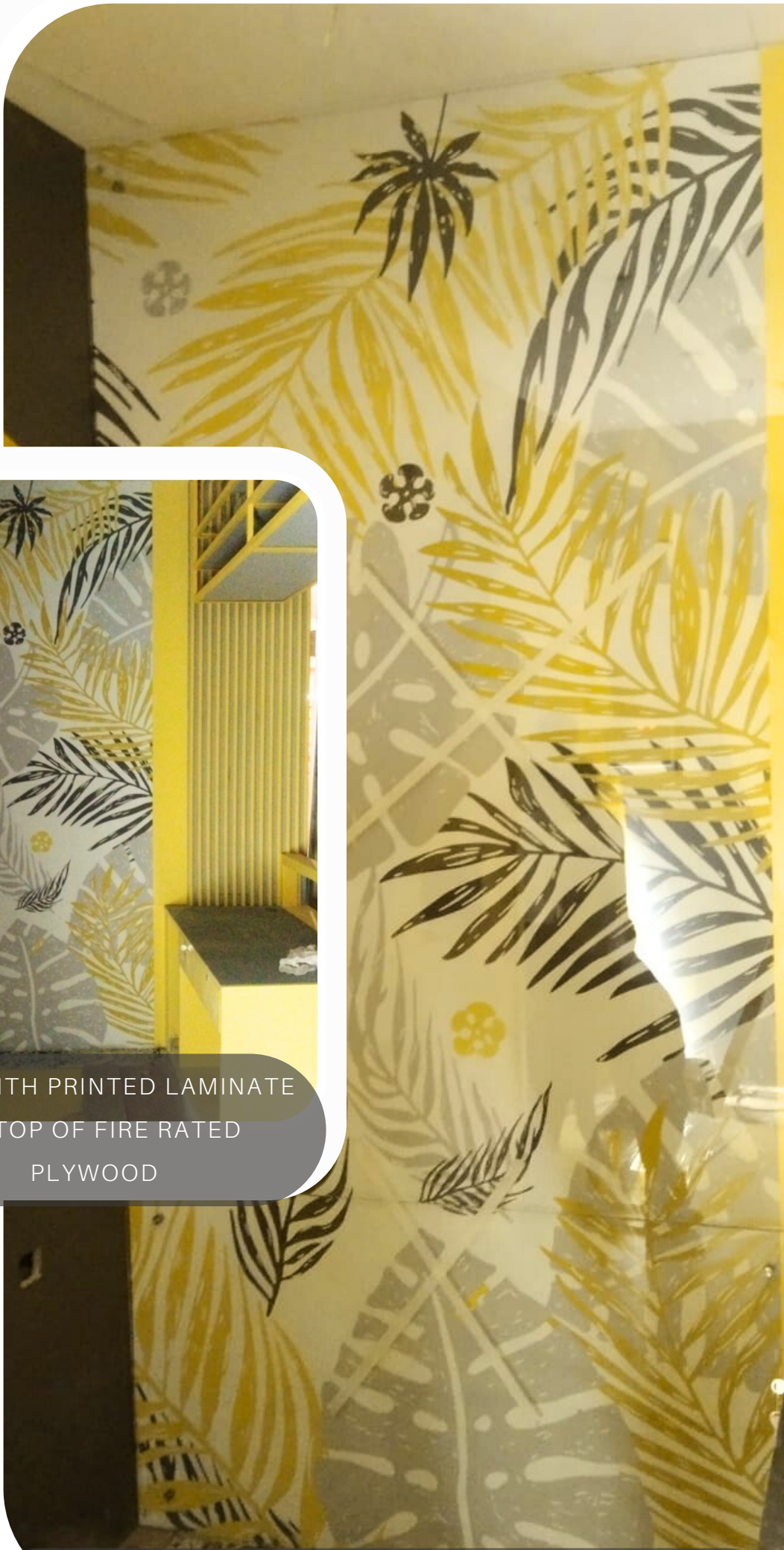
FINAL LOOK OF SIDE WALL B WITH GLASS MOUNTED ON TOP
