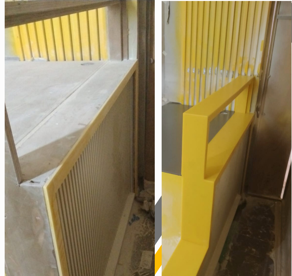
COUNTER FACIA UNDER PROGRESS - PLY CUT INTO REQUIRED PROPORTIONS ALONG WITH FLUTED PIPES AND SURFACE FINISHED WITH SPRAY PAINT OF CHOSEN COLOR AFTER FIXED
