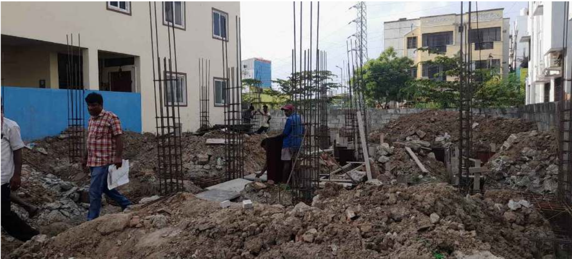
SITE VISIT ON 27.04.2023 INSPECTION ON PILE CAP REINFORCEMENT, PLINTH BEAM REINFORCEMENT, SHUTTERING AND COLUMN ALIGNMENT
