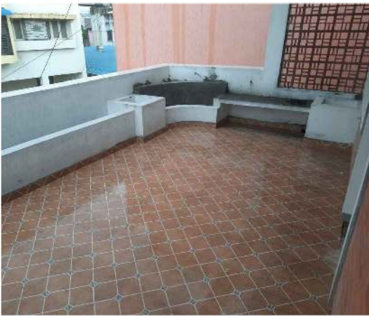
SITE VIEWS OF TERRACE GARDEN
