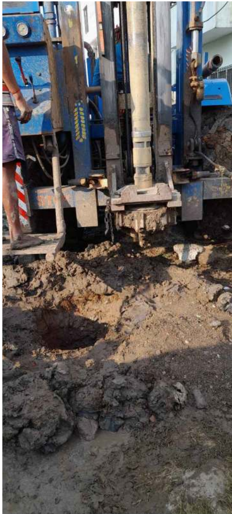
SITE VISIT ON 13.03.2023 INSPECTION ON PILE FOUNDATION LAYING PROCESS
