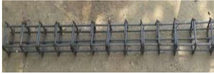
Fig 4.14 Reinforcement of RC beam
