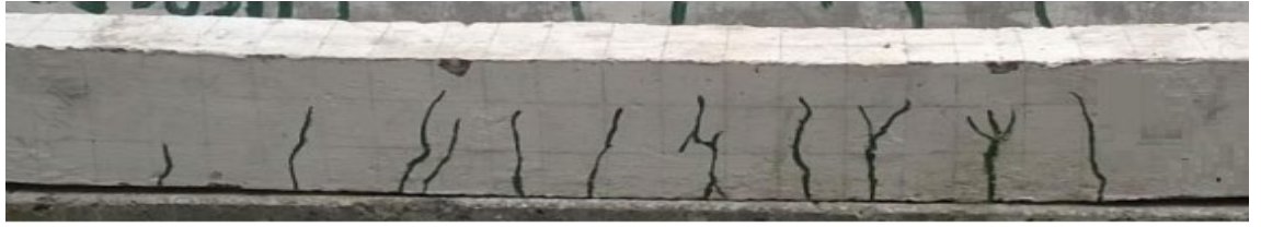
Fig 4.17 Crack pattern of specimen
