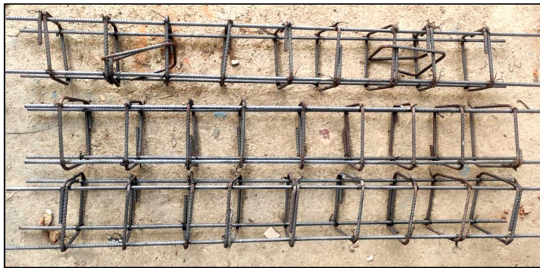
Fig 4.15 Reinforcement for beams
