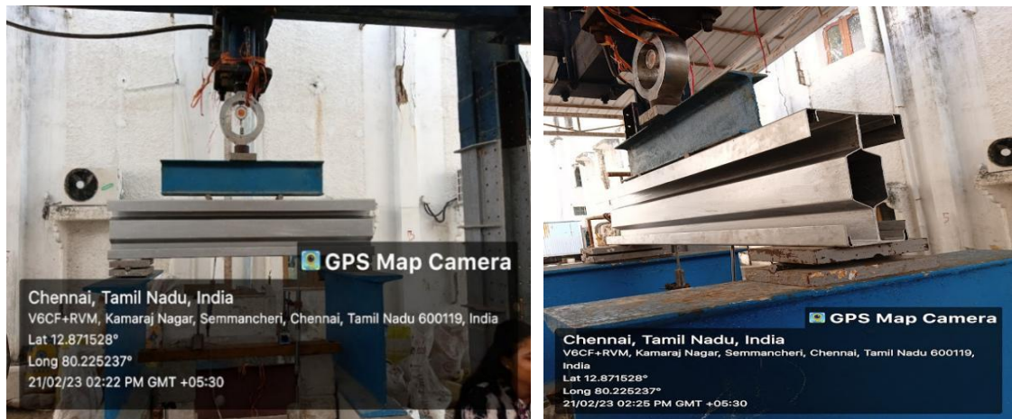
Fig 4.7: MSBB Before Applying Load
