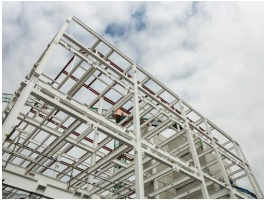
Fig. 1.2 Cold-Formed Steel Structure
