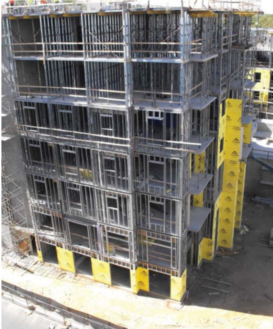
Fig. 1.1 Cold Formed Steel Building
