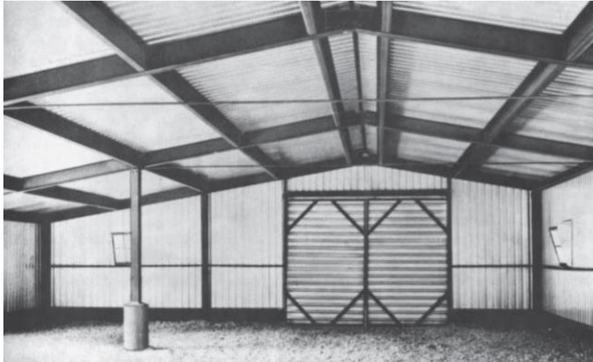
Fig. 3.4 Structure of cold-formed steel
