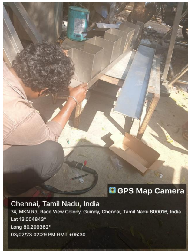
Fig 3.6: Welding of cr2 steel sheet
