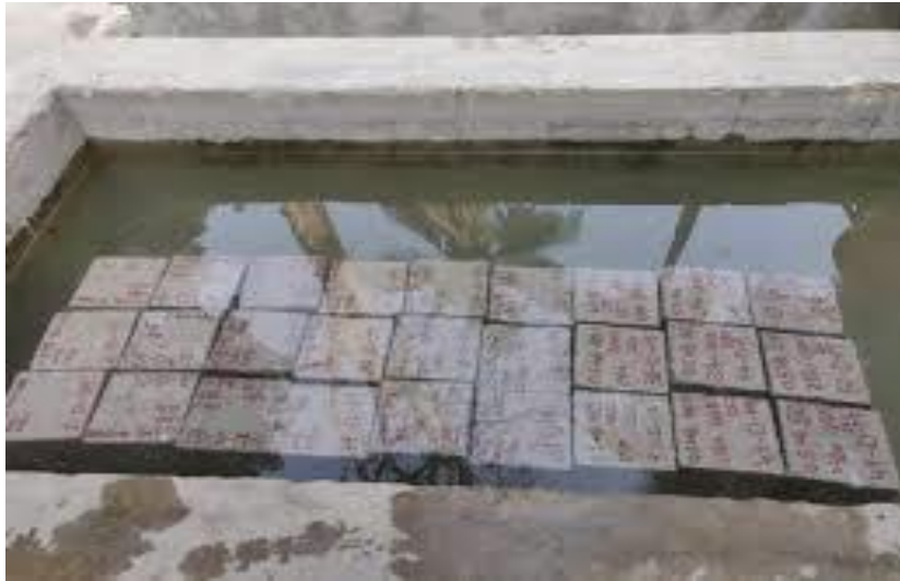
Fig 3.10: Curing of concrete
