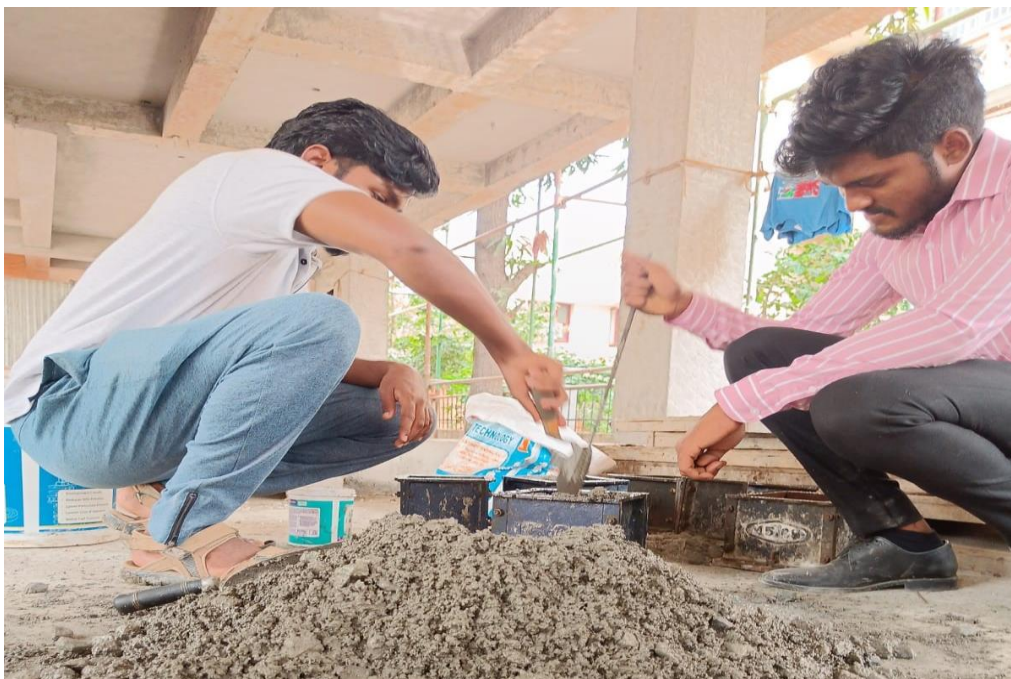
Figure 4.2: Mixing of Concrete
