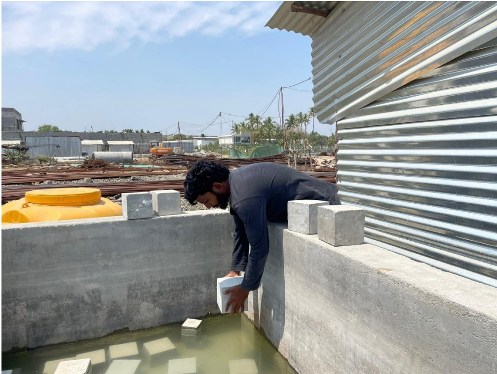
Figure 4.5: curing concrete cubes
