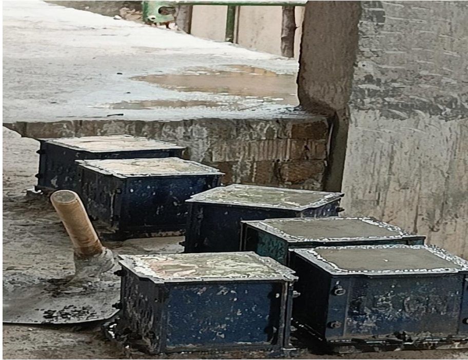
Figure 4.13: Prepared concrete mould
