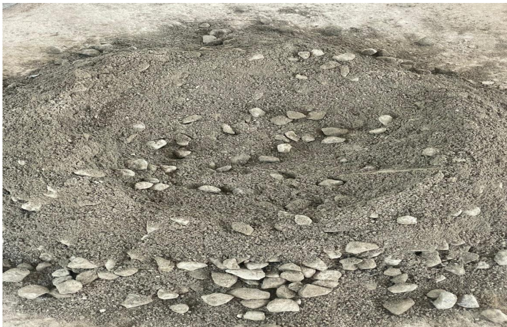
Figure 4.9: Mixing of mortar
