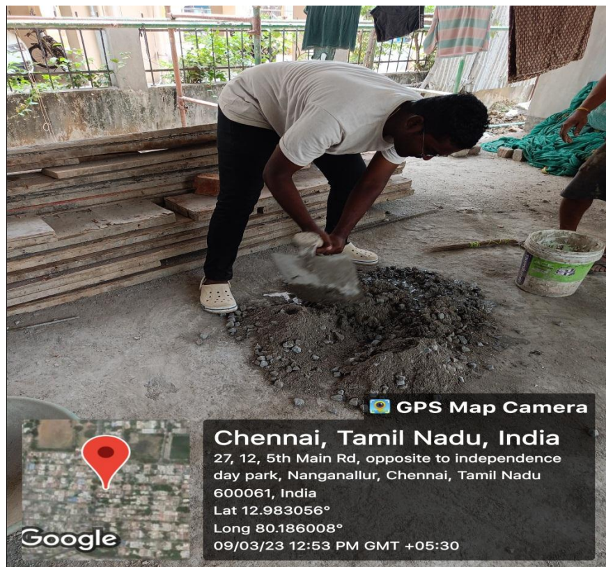
Figure 4.10: Mixing of concrete
