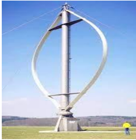
Fig.1.6 Darrieus type Vertical Axis Wind Turbines
