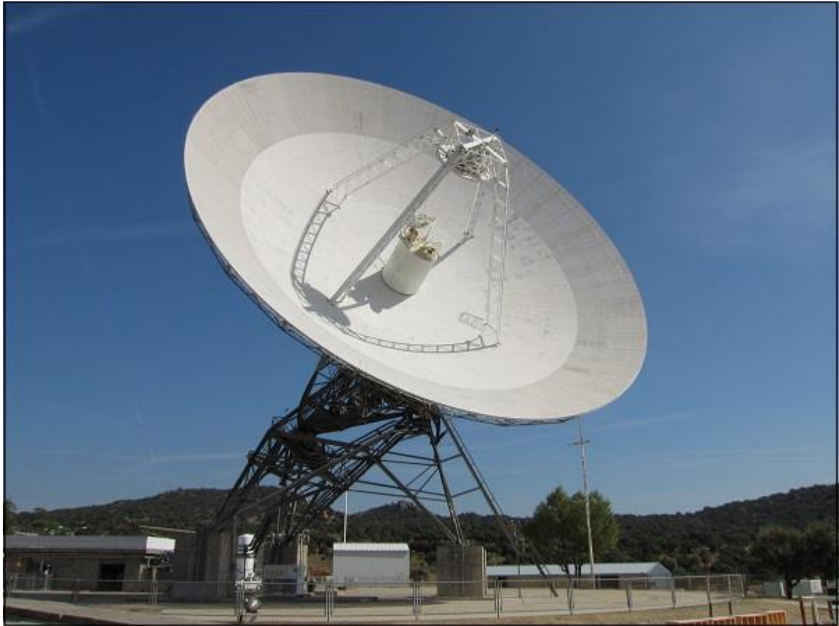
Fig:15 paraboloid reflector with cassegrain feed
