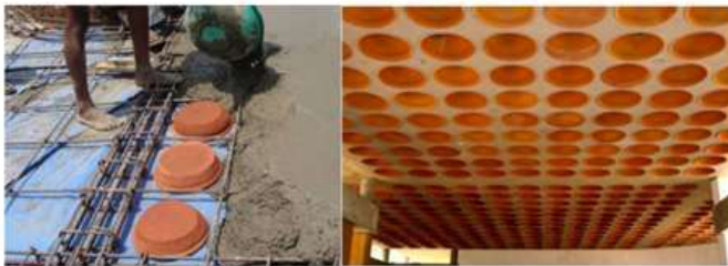
Fig.15. Filler slab with terracotta pans
