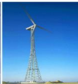
Wind Turbine - Lattice Tower
