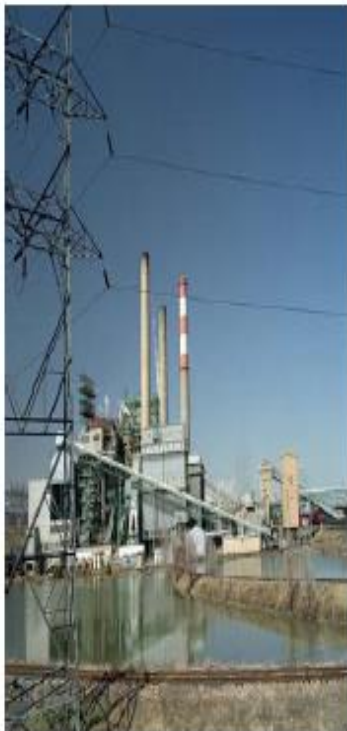
Central Power Plant
