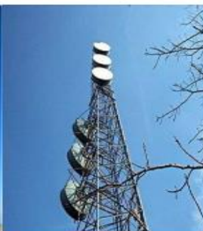
Radio Lattice Tower
