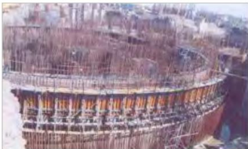
Fig.3- IC Wall Construction in progress
