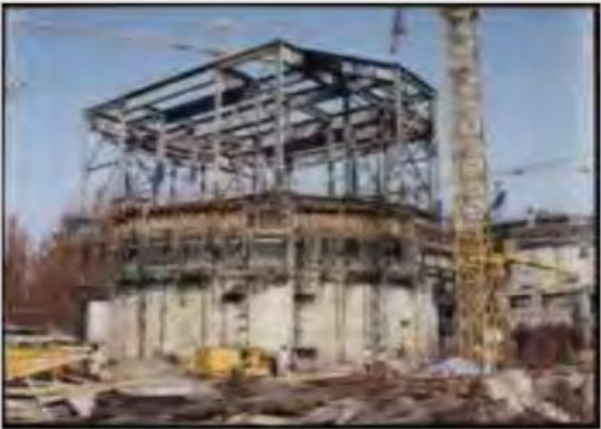
Fig.4 -Reactor building internals- structural steel framework
