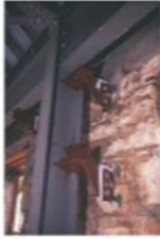
Figure 8: Adding new member for Strengthening
