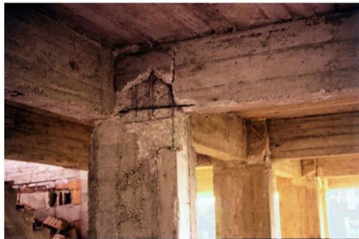
Figure 2: Spalling of Concrete at Joints
