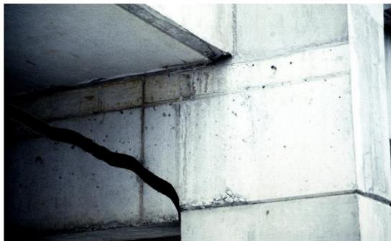
Figure 3: Diagonal Cracks at joints
