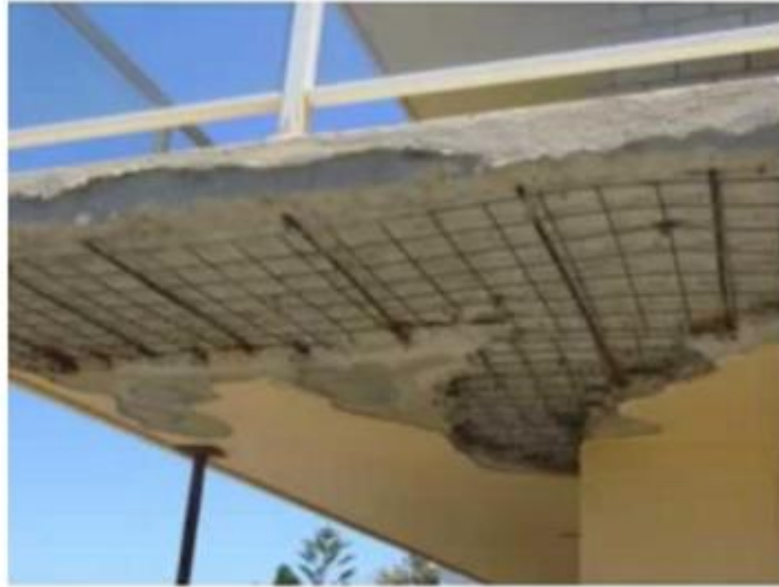
Figure 1: Spalling of Concrete
