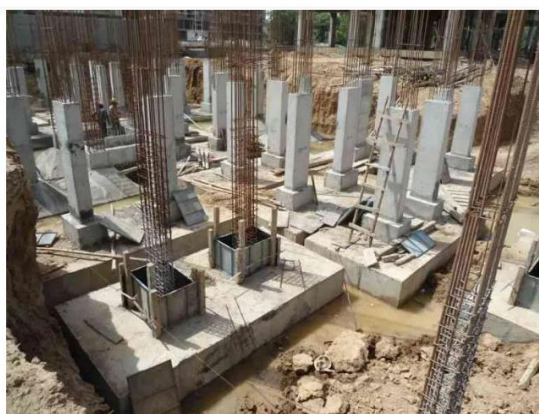
Fig 2 Combined Column Footing
