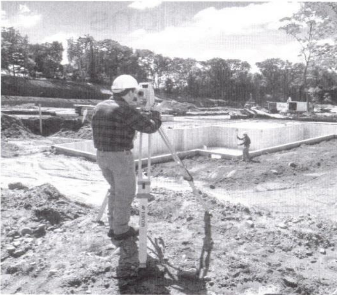
Measuring with a total station
