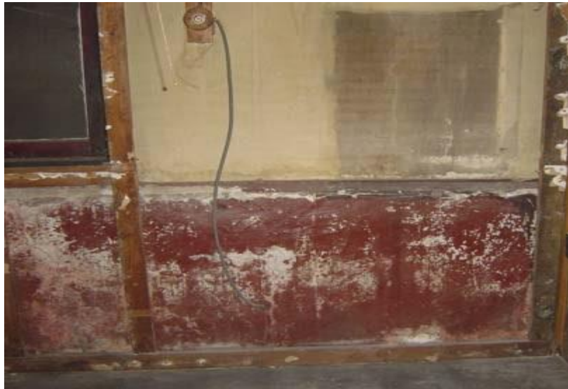
FIG.17 EFFLORESCENCE
