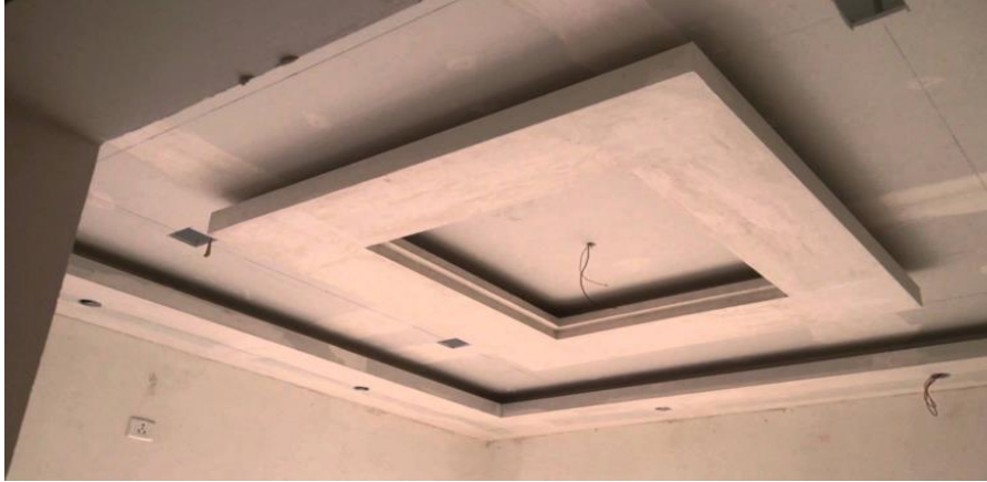
FIG. 3 GYPSUM BOARD FALSE CEILING
