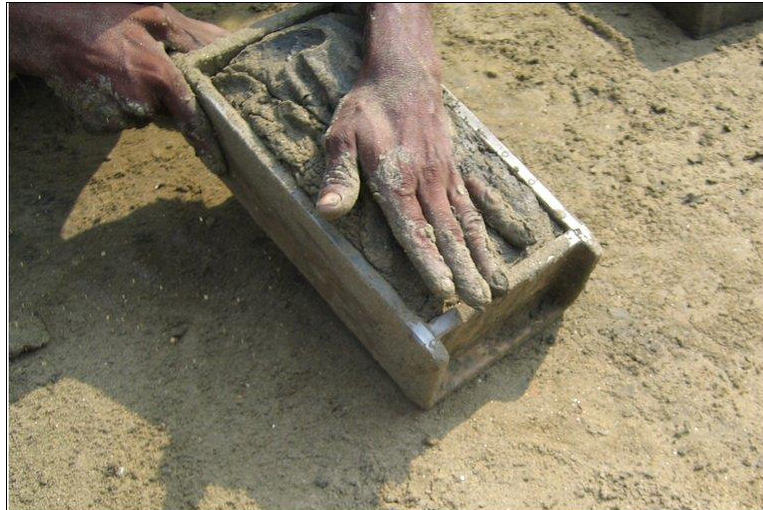
FIG.11 HAND MOULDING OF BRICKS
