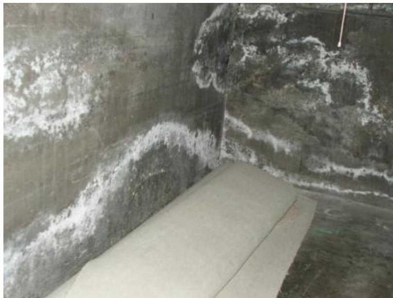
FIG.17 EFFLORESCENCE ON PLASTER
