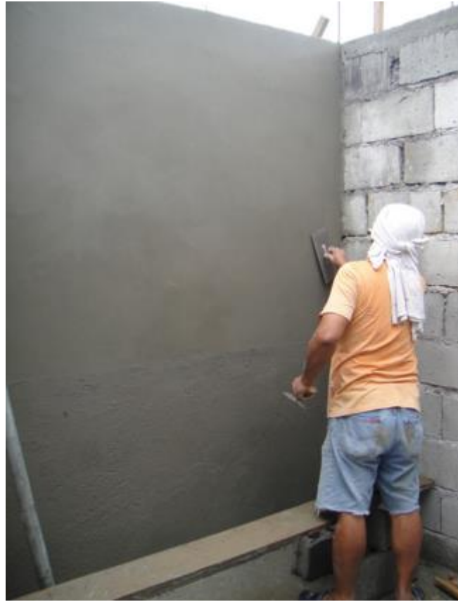
FIG.31 WALL CEMENT MORTAR PLASTERING
