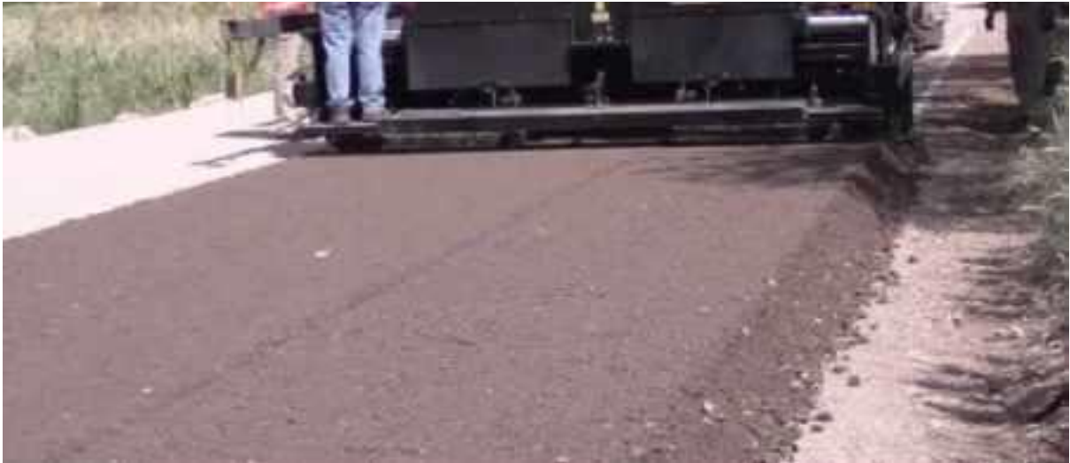
Fig. 4 Providing Base Course
