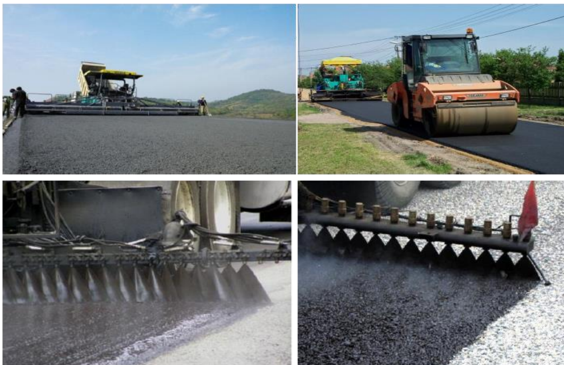
Fig 10 Construction procedure of flexible pavement
