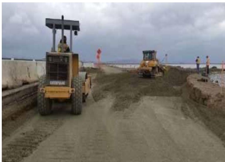
Fig. 5 Laying of Subbase Course
