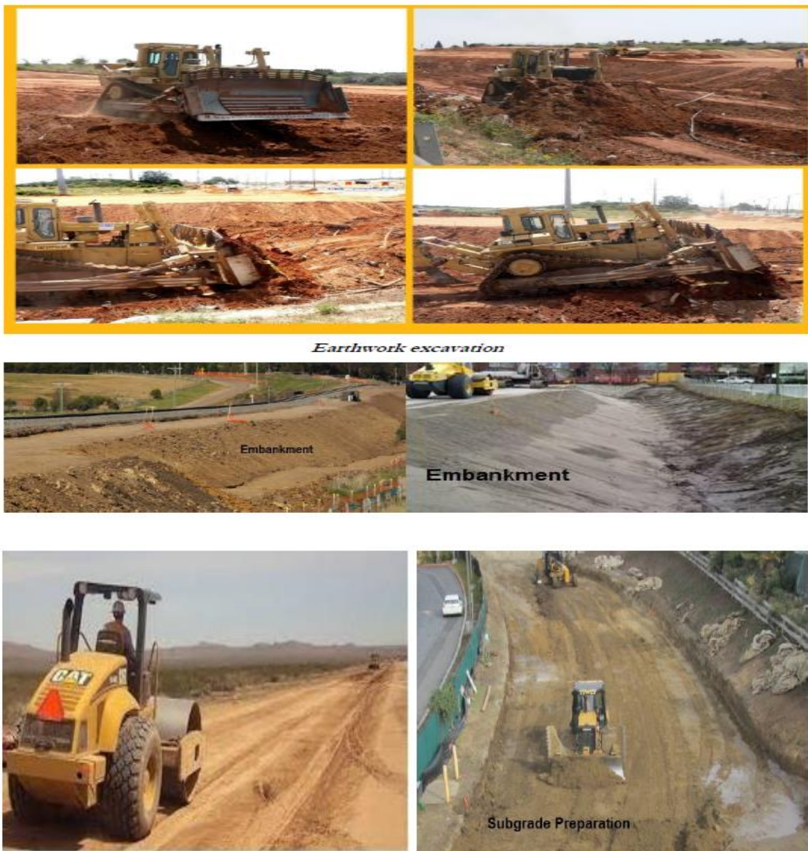
Fig 9 Construction phase of flexible pavement
