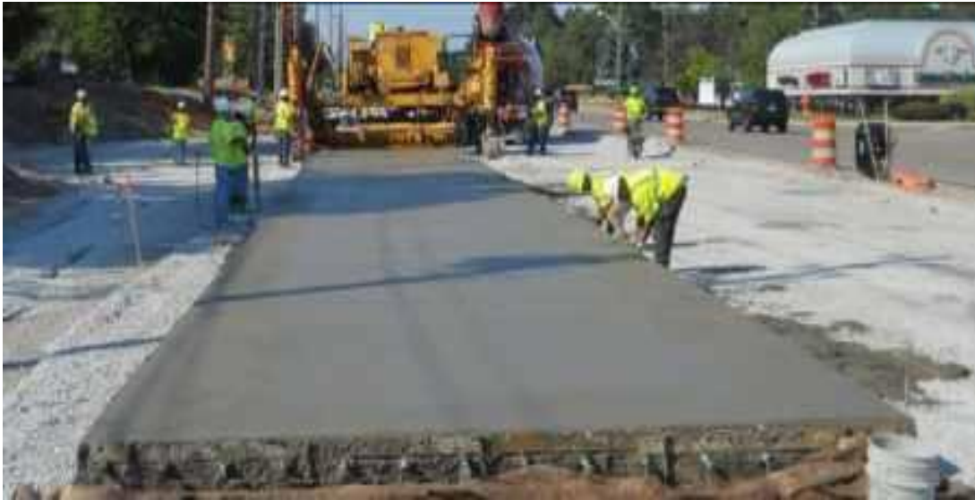
Fig. 3 Concrete Slab Laying
