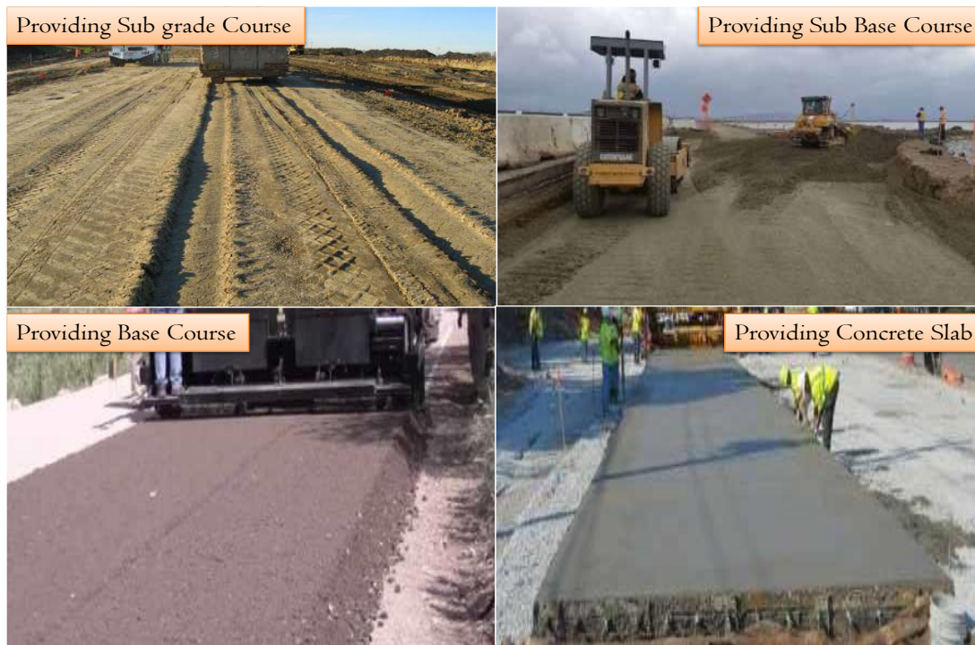
Figure No.6 Layers of rigid pavement
