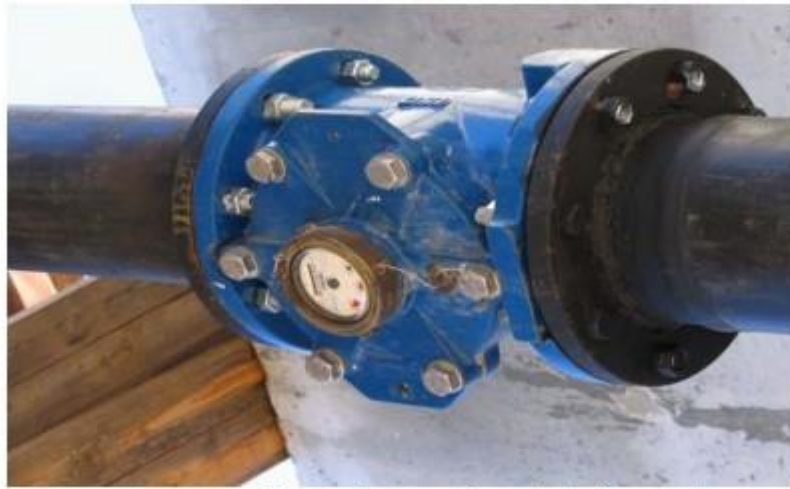
Measuring pumping rate by flow meter
