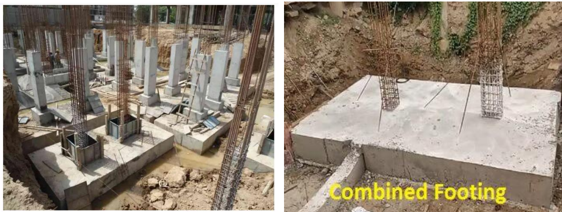
Fig 2 Combined Column Footing
