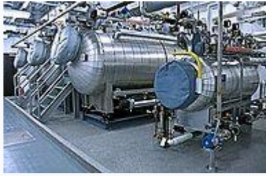
Effluent decontamination system of a BSL-4 lab of NIAID
