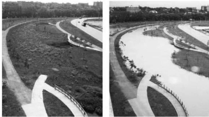
The lower spreading basins closest to the river are shown during both a dryer period on left and following a heavy rainfall on right, illustrating the site's flexibility and multipurpose capacity.
