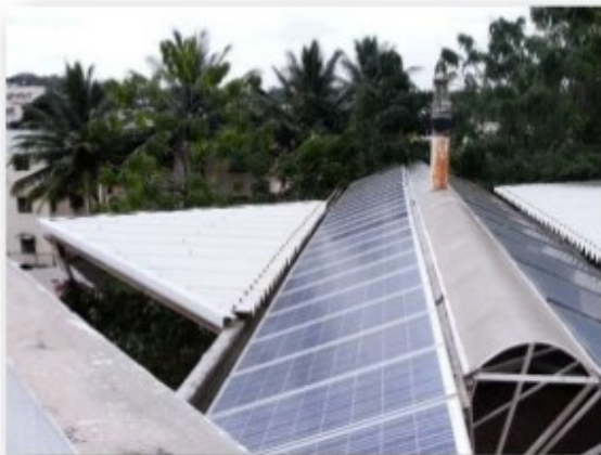
Solar Photovoltaic integrated with the roof provide natural light and electricity
