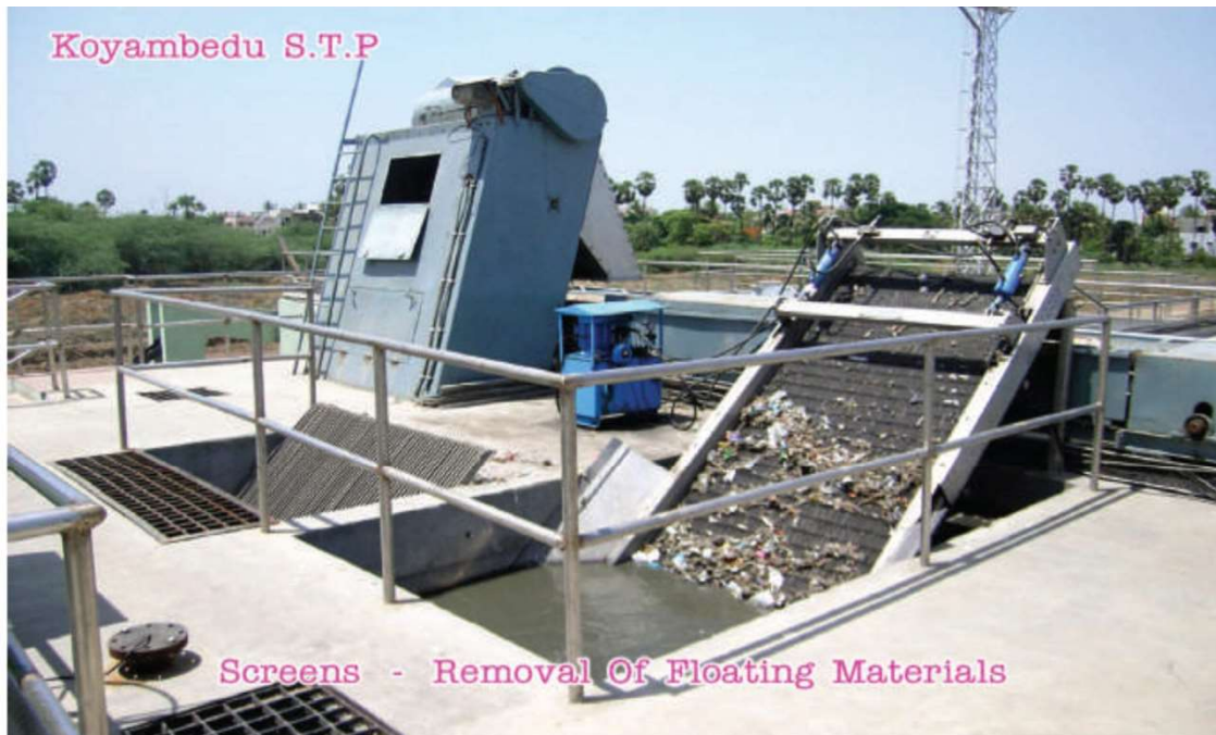
Mechanical screen with screen housing and ventilation at Koyambedu STP in Chennai. Manual screen and bypass channel screen in between the mechanical and manual screens is also seen
