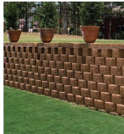
Figure 1.27 Screen block retaining wall
