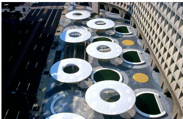
Figure 1.15: Hud Plaza, Washington, USA
