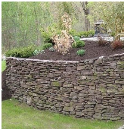
Figure 1.26 Stone retaining wall
